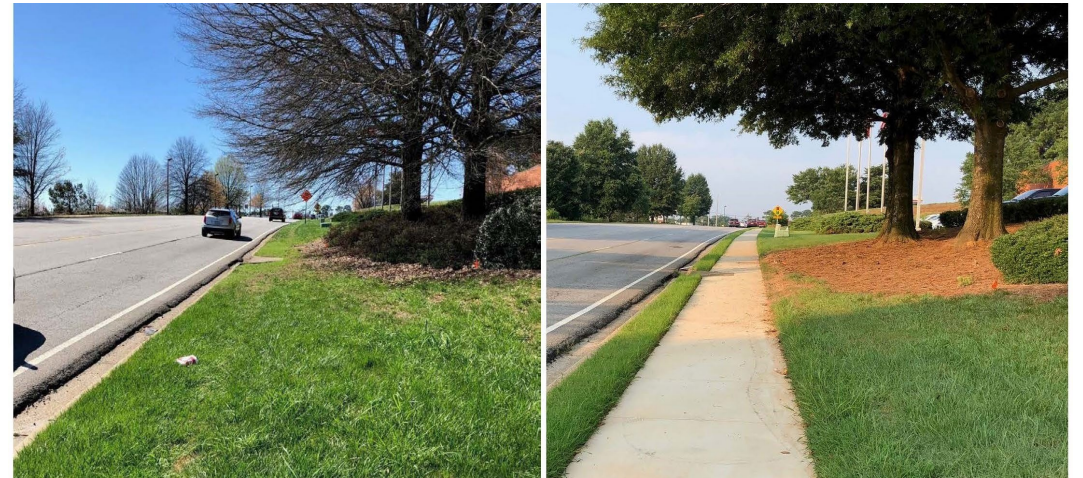
Three sidewalk projects completed with SPLOST funds
