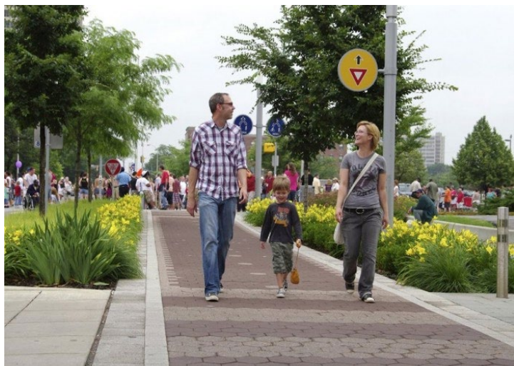
The trail incorporated pavers and landscape buffers into the design. (Source: indyculturaltrail.org )
