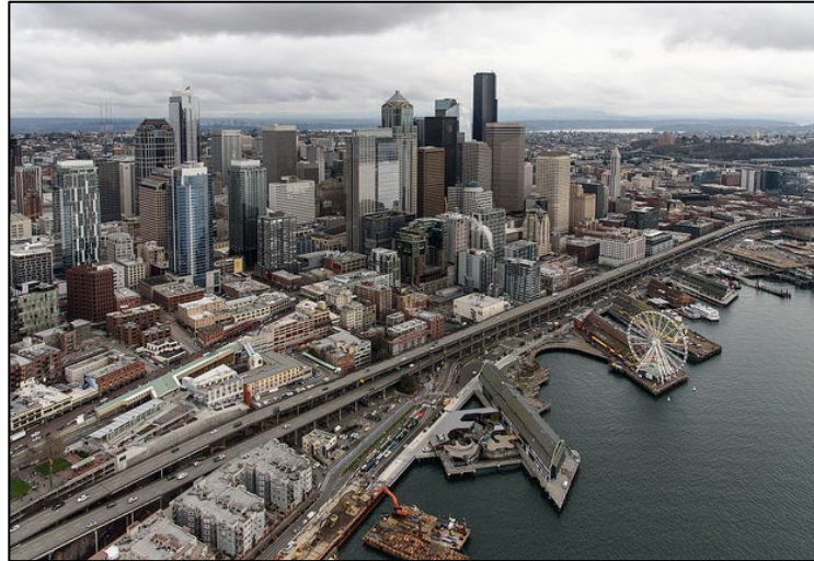
This is an aerial view of the Alaskan Way Viaduct prior to demolition. (Source: WSDOT)
