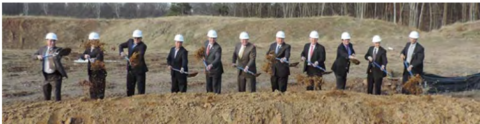
Pacific Boulevard Ground Breaking: Route 28
