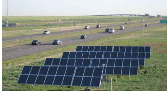
E-470 solar array.
