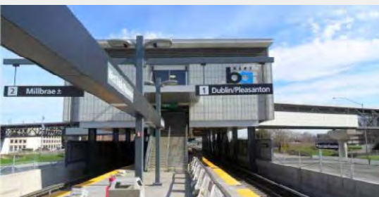
West Dublin/Pleasanton Station.
