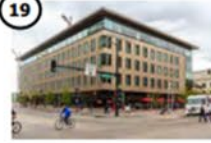
S. WING BUILDING ONE UNION STATION (2014) 5 Story Office, Retail
