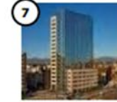
1900 16 th STREET (2009) 17 Story Office, Retail & Living Space
