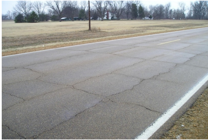
Figure 1. Example of block cracking from age-related embrittlement.
