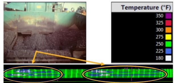
**Figure 2. Effects of running the paver hopper low on the thermal profile.**
