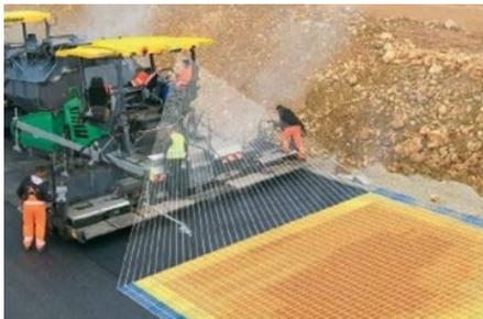
**Figure 1. PMTP system measuring thermal profiles behind the paver.**
