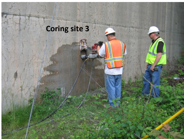
Figure B1: I395 over Main Street
