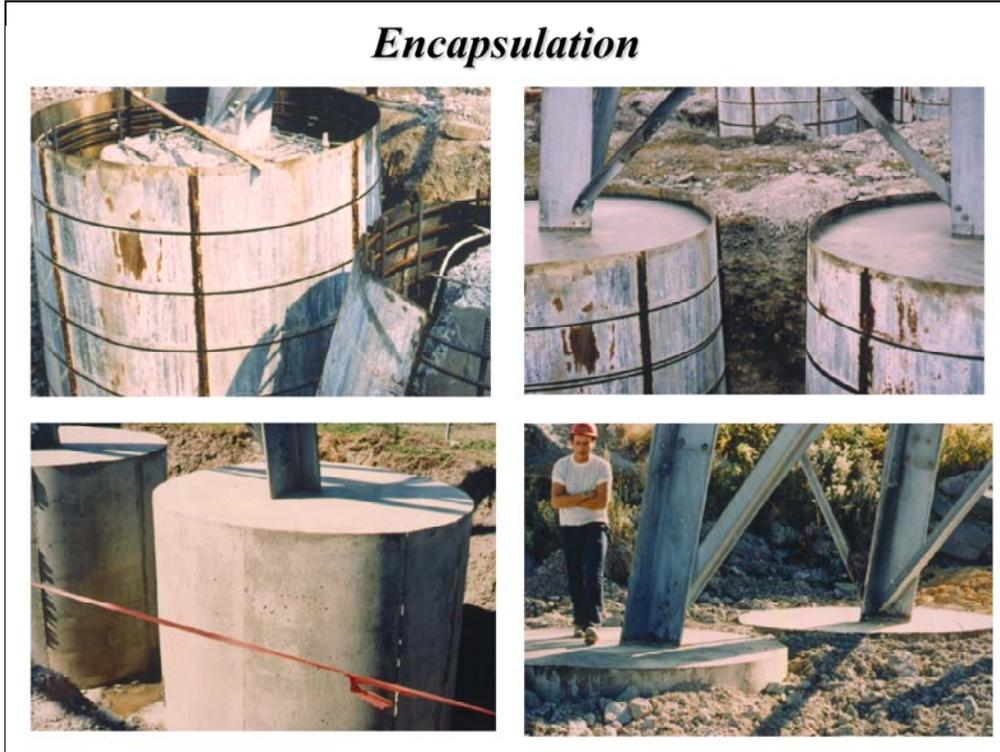
This slide shows the placement of external formwork around the footings, on top, and the final product, on the bottom, once the forms were removed.
