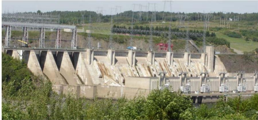
Aggregate passed ASTM C 227 – “non-reactive”
