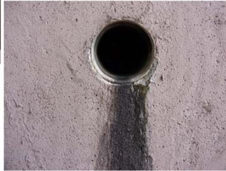
Improving the drainage of water away from ASR-affected structures is a simple, yet effective, method of reducing the internal relative humidity in concrete.
