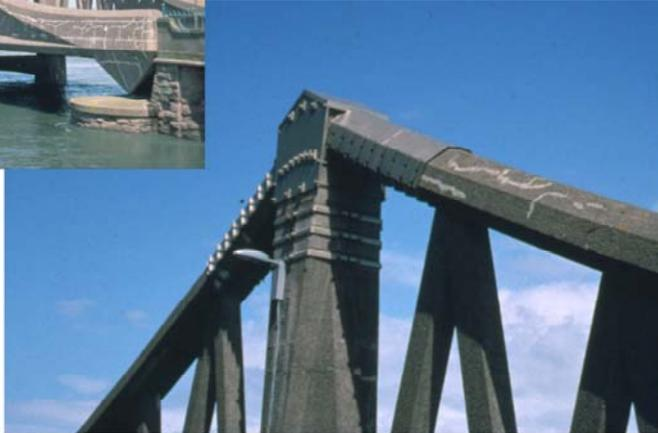
These photographs show another case study where external, physical restraint was applied to attempt to mitigate the effects of ASR damage in this arch bridge in Scotland.
