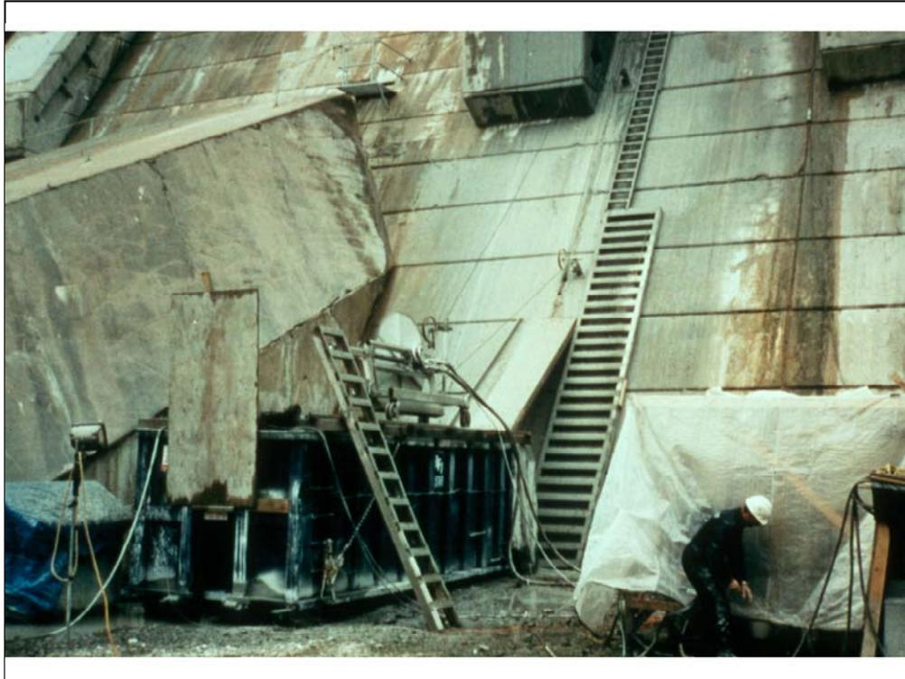
This photograph shows the equipment used for “slot cutting.” The procedure itself is not fancy, but it is effective.
