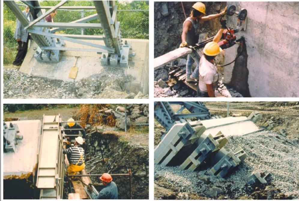
Some of the damaged footings were also post-tensioned, as part of the repair regime. This post-tensioning was passed through the original footing and anchored and tensioned to provide active restraint.
