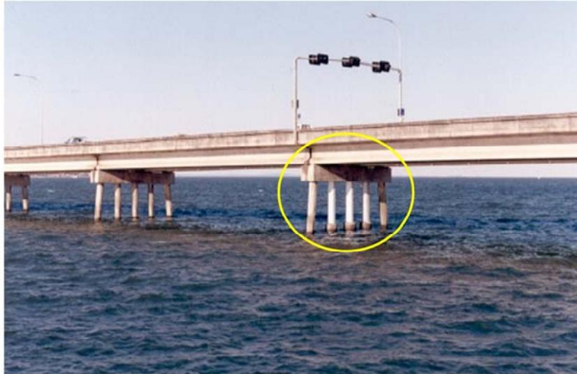
Bridge structure affected by ASR in Brisbane, Australia. The piles were wrapped with composite materials. The piles selected to be repaired by this method were those in which the ASR process was almost completed. It was also selected to try to minimize further deterioration due to corrosion (exposure to marine environment)
