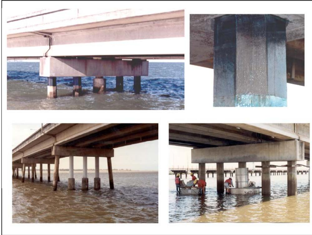
This slide shows the application of FRP wraps as a form of external restraint to ASR-affected columns. Again, this example is from a bridge in Australia.
