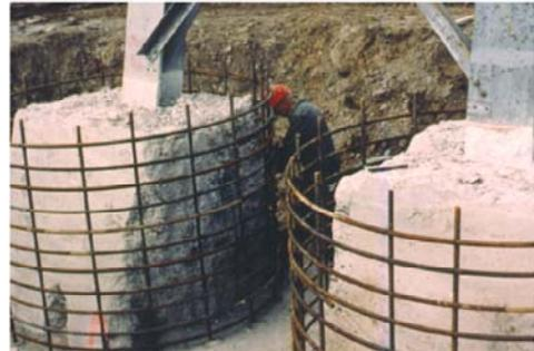
These photos show the removal of the damaged concrete and the placement of the rebar cage (around original footing).
