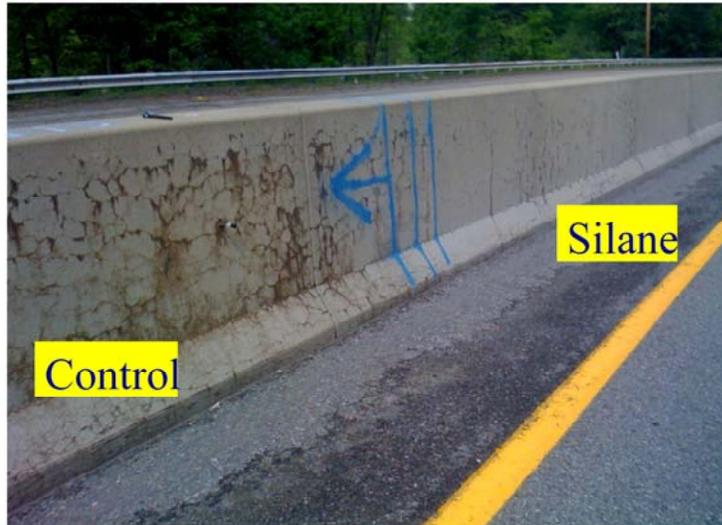
Coming back to the application of silanes under the FHWA project in Massachusetts, one can see that there is once again an obvious difference in the visual appearance of silane-treated and untreated barriers four years after treatment. Long-term monitoring has confirmed that the internal relative humidity has been reduced significantly for the silane-treated barriers.
