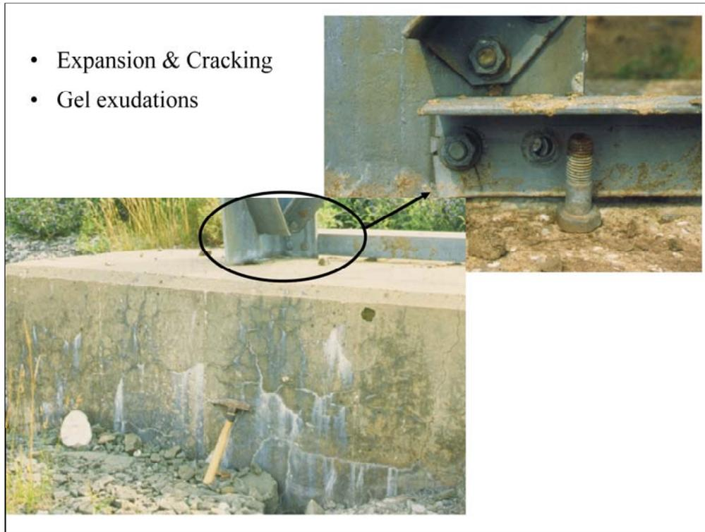
This slides shows a couple photographs showing the symptoms of ASR within these footings, prior to repair.
