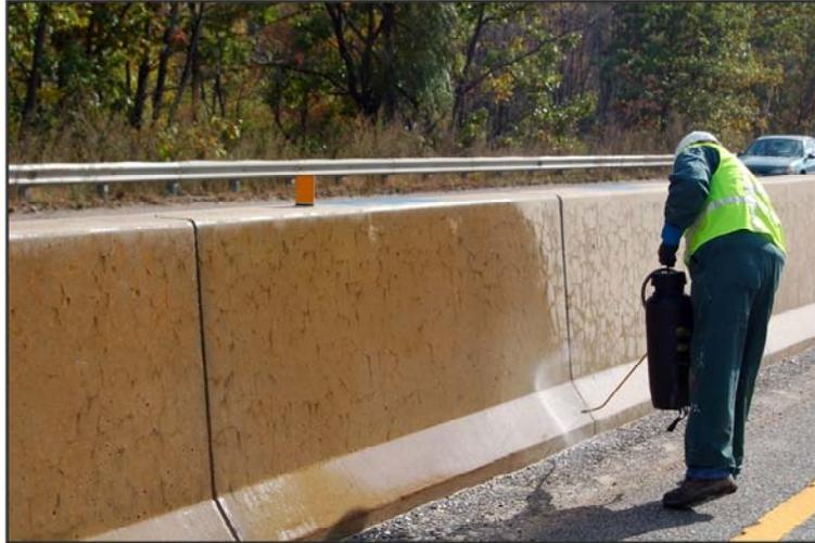
This photograph shows FHWA researchers applying a 30% lithium nitrate solution topically to the barriers in Leominster, MA.
