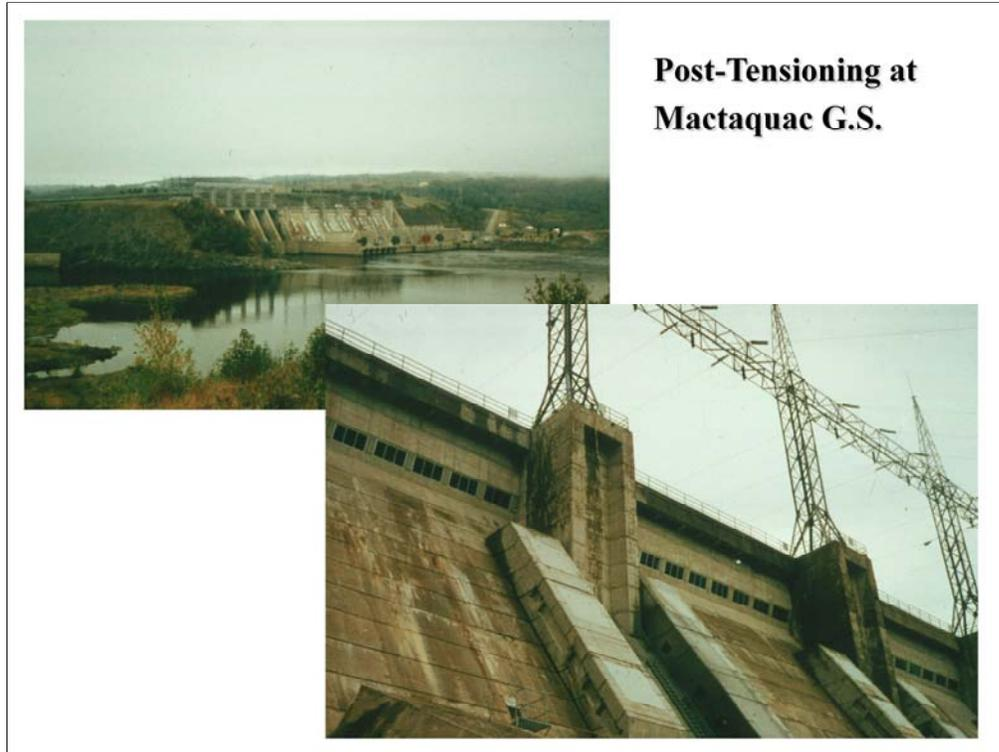
Another interesting case study related to providing external (or internal) restraint is the Mactaquac Dam in New Brunswick, Canada. This dam has been suffering from ASR for quite a few years, and for a time, there was concern about some larger cracks that could affect the structural performance and safety of the dam. Post-tensioning was selected as a methodology for this dam, as discussed next.
