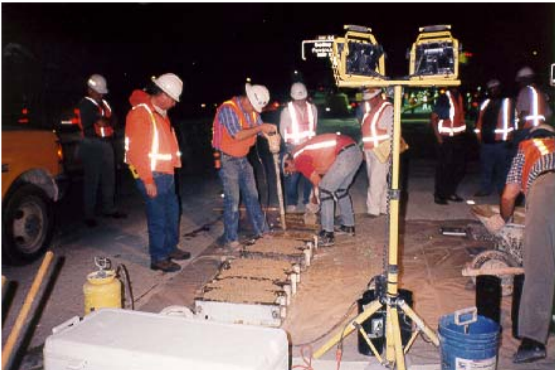
Photo 3: Beams being cast
