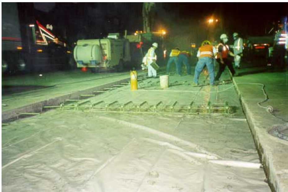
Photo 1: Dowel bars and tie bars are being placed
