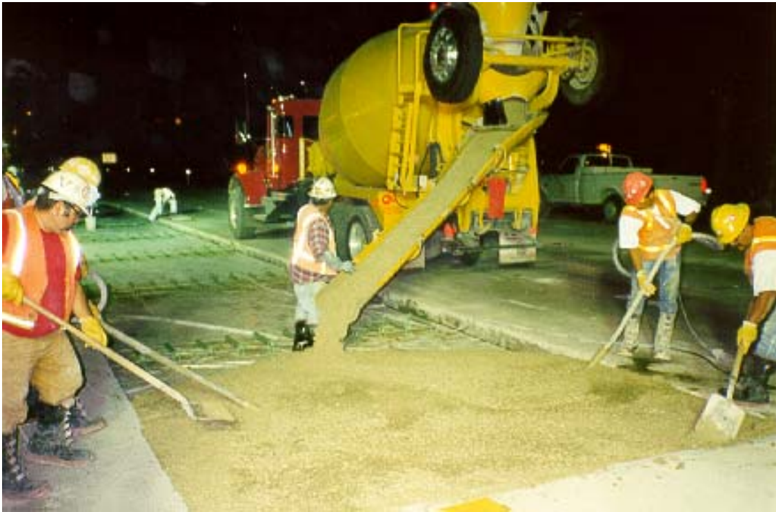
Photo 2: FSHCC being placed
