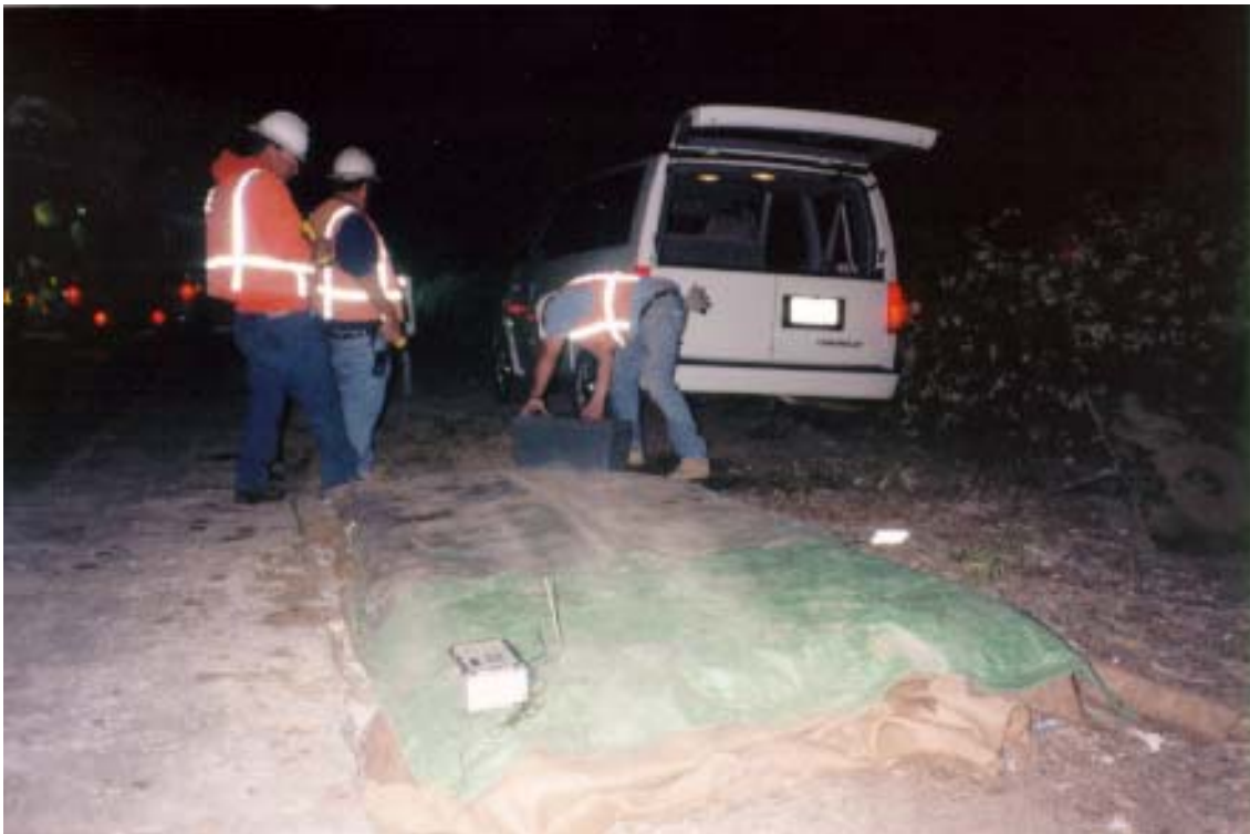
Photo 4: Beams and cylinders being covered during initial curing
