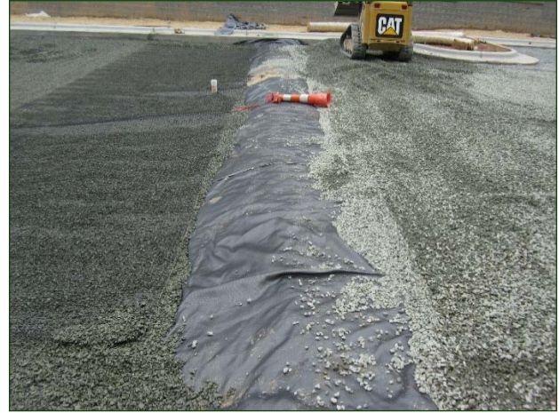
Figure 12. Aggregate and impermeable liner flow barrier
