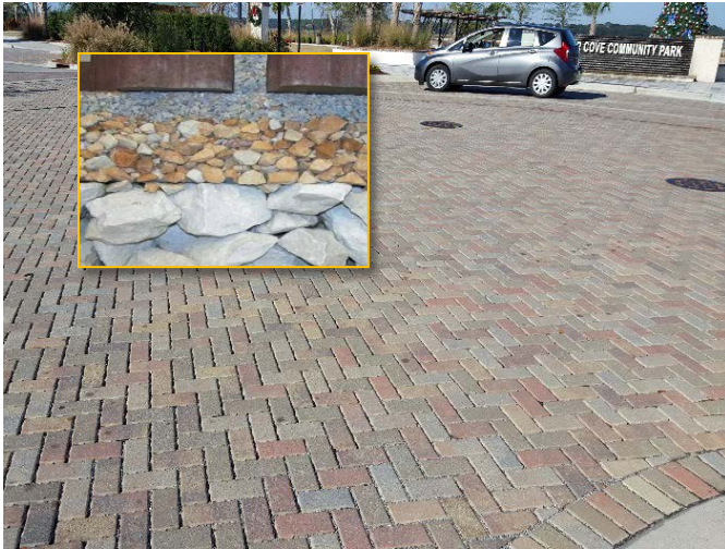
Figure 2. Photo. Permeable interlocking concrete pavement – Hilton Head, South Carolina
