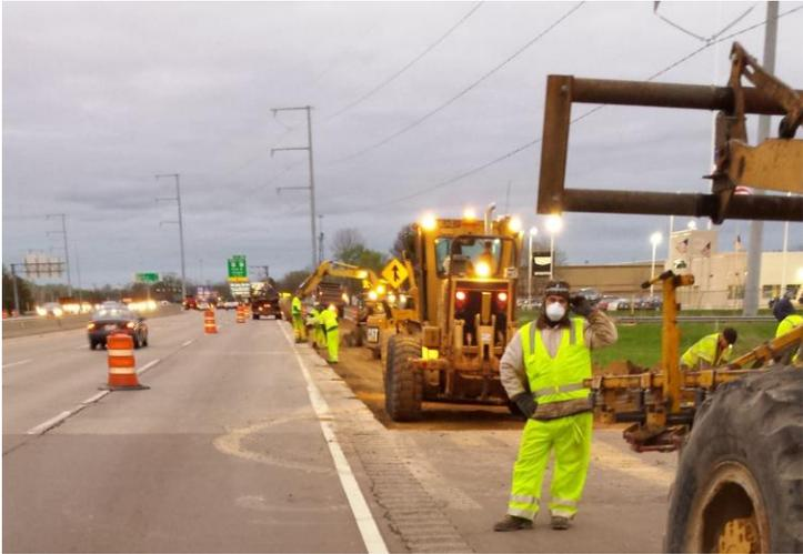
Figure 9. Photo. Stage 1 lane closure and traffic flow.
