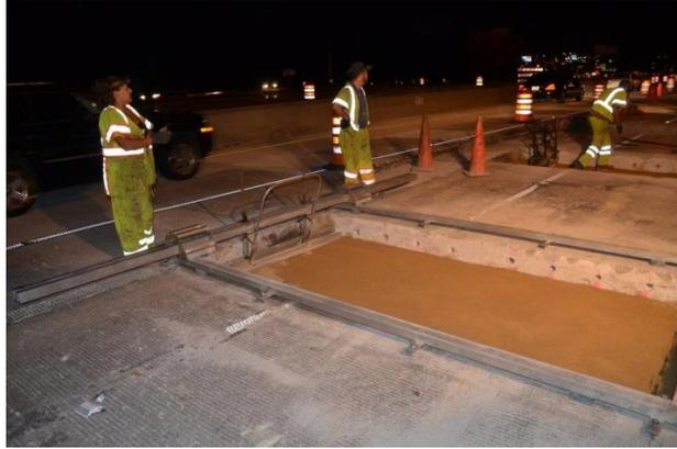
Figure 18. Photo. Fine-grading of the bedding layer.
