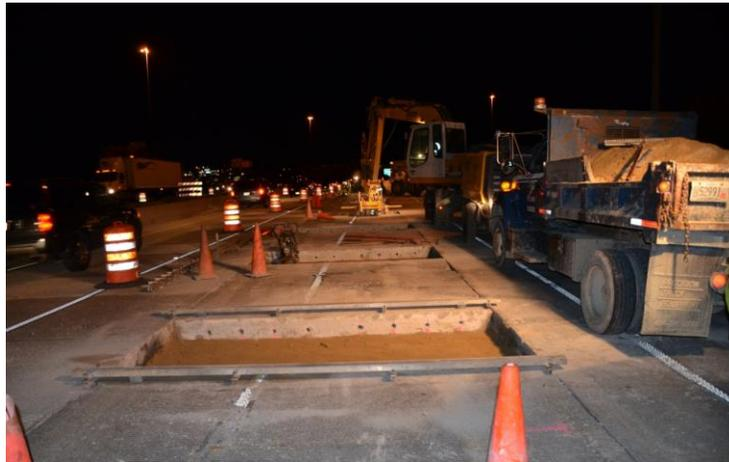
Figure 16. Photo. Distressed slab removal process.
