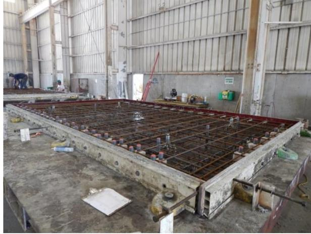
Figure 3. Photo. Super Slab panel form setup.
