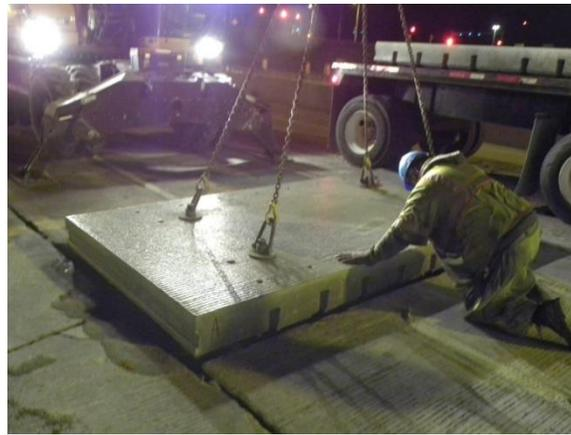
Figure 21. Photo. A typical panel placement.
