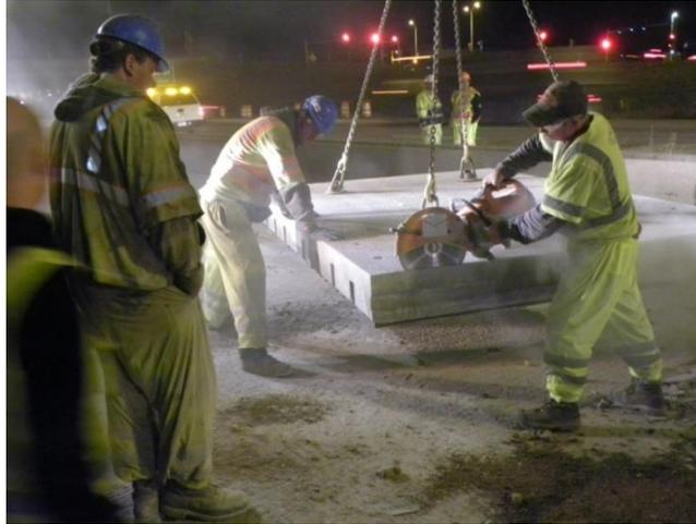
Figure 20. Photo. Panel trimming operation.
