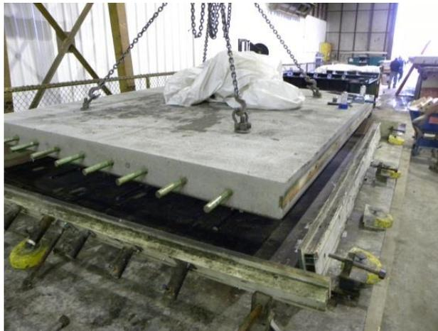
Figure 4. Photo. Super Slab panel form stripping.
