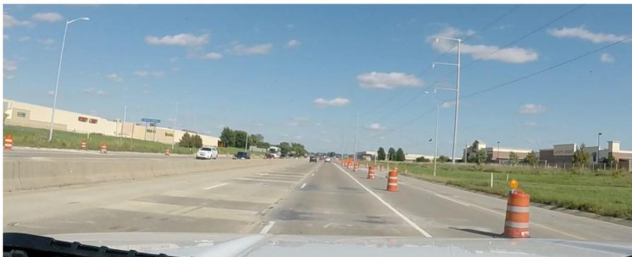
Figure 13. Photo. Stage 3 outside shoulder closure and traffic flow after completed repairs in Lane 2 and Lane 3.
