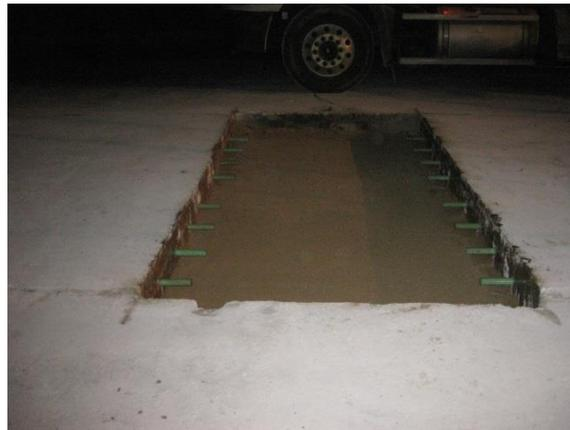
Figure 17. Photo. Dowel bars installed in the repair area.
