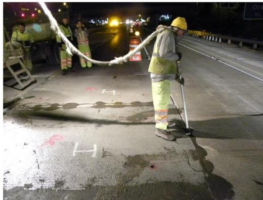
Figure 23. Photo. Grout application along a longitudinal joint.
