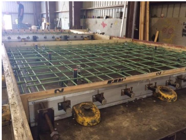
Figure 11. Photo. Panel formwork setup.
