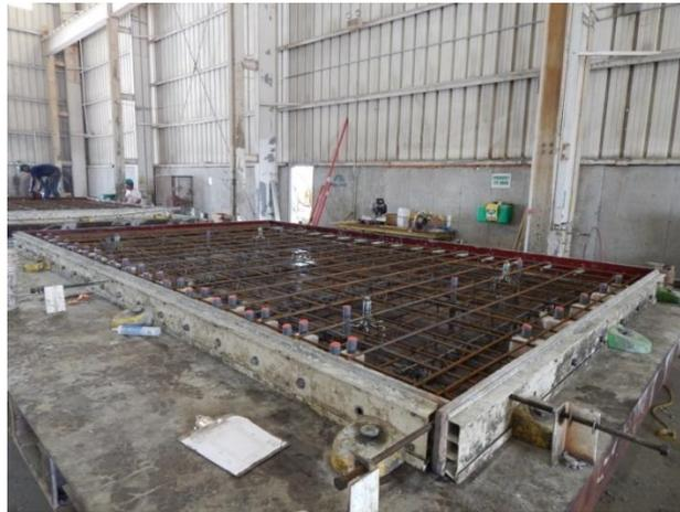
Figure 6. Photo. Super Slab panel form setup
