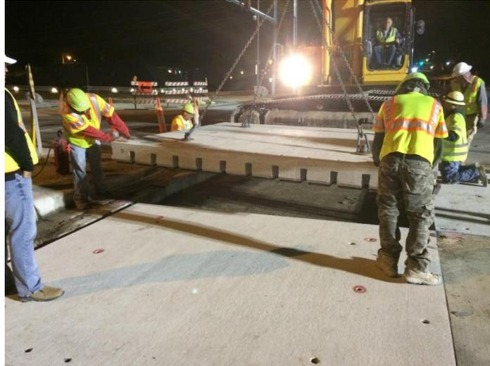
Figure 17. Photo. A typical panel placement.
