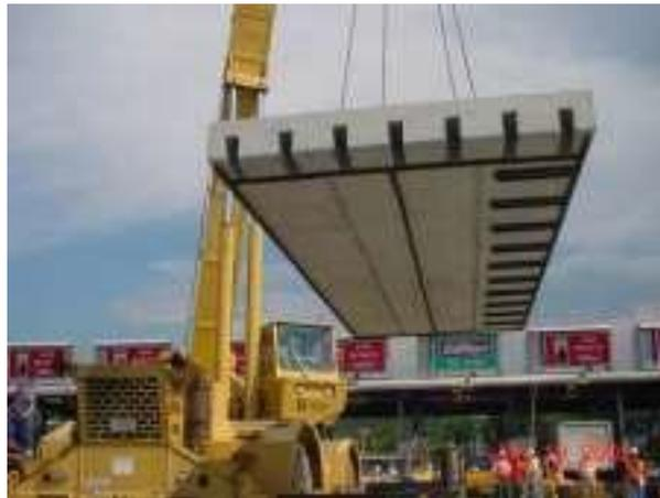
Figure 8. Photo. Dowel bar slots and foam gaskets at the panel bottom.
