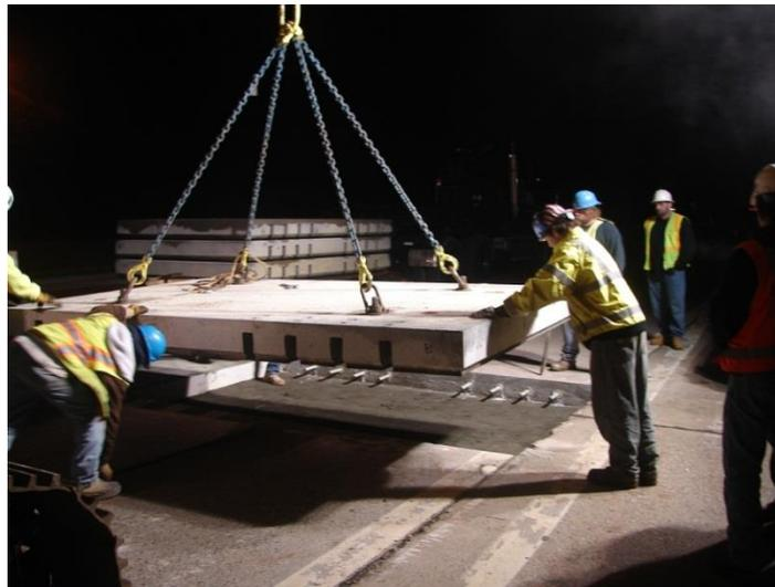
Figure 10. Photo. Super Slab system panel installation.
