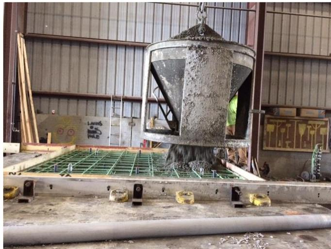
Figure 13. Photo. Concrete placement in the panel formwork.
