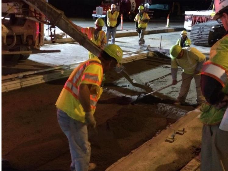
Figure 15. Photo. Placement of the cemented bedding layer.
