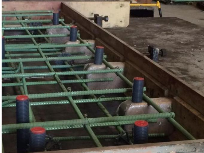
Figure 12. Photo. Close-up view of the panel formwork setup.
