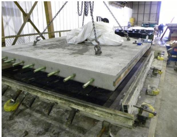
Figure 7. Photo. Super Slab panel form stripping.
