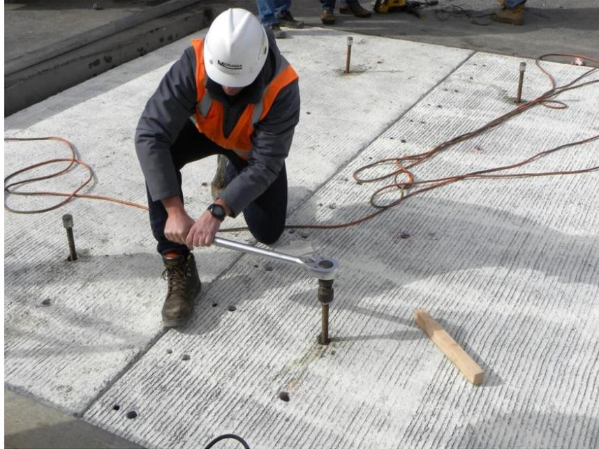
Figure 20. Photo. Using leveling bolts to set panel elevation.
