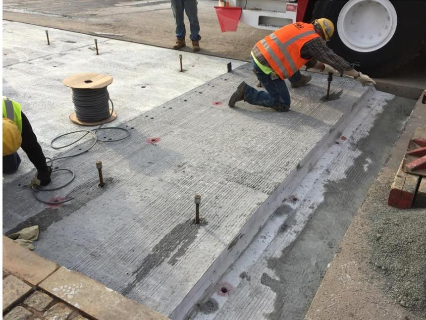
Figure 22. Photo. Transition panel installation at the north bus pad.
