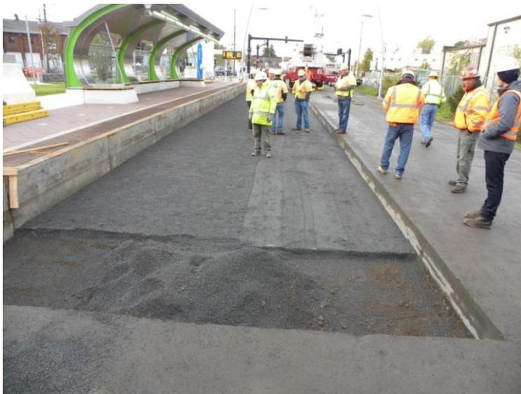
Figure 15. Photo. Removal of about 6 feet of the bedding layer at the north bus pad end.
