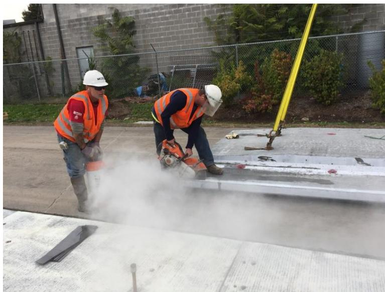
Figure 21. Photo. Trimming the transition panel at the north bus pad.
