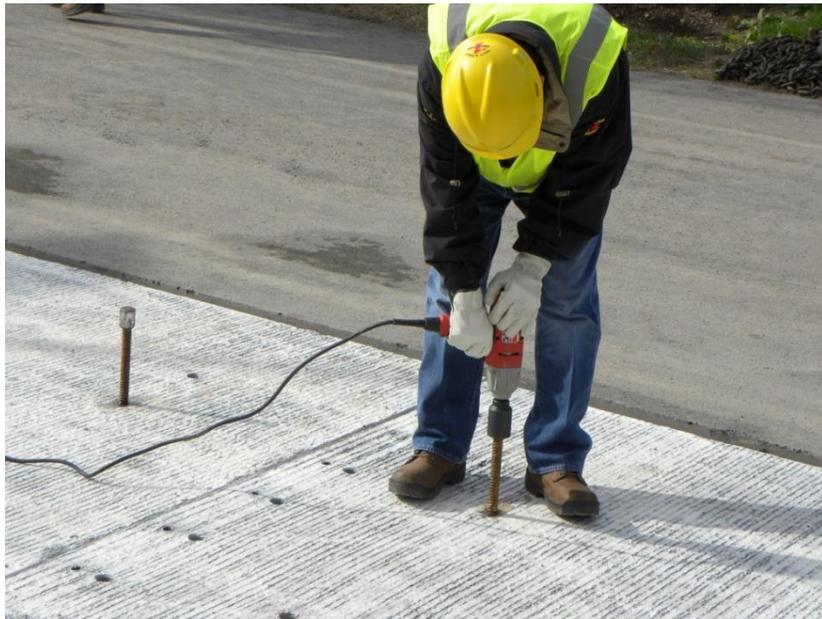
Figure 19. Photo. Separating the leveling lift plate from panel bottom.
