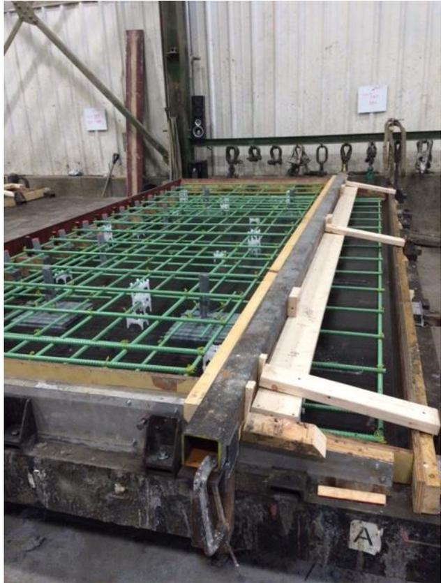
Figure 9. Photo. Transition panel formwork setup.
