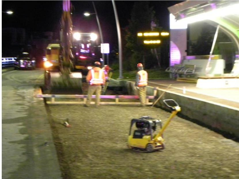
Figure 12. Photo. Open-graded bedding layer placement at the north bus pad.
