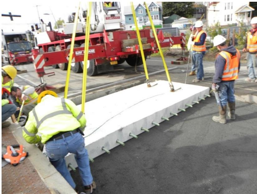
Figure 17. Photo. Placement of the first panel at the north bus pad.
