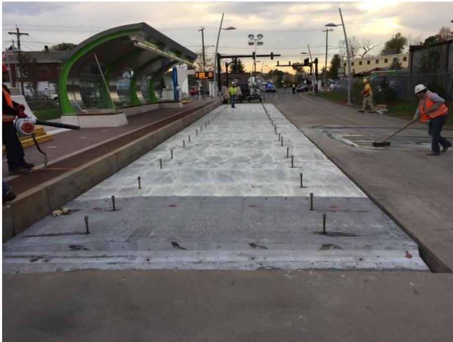
Figure 23. Photo. Panels with leveling lifts engaged at the north bus pad.
