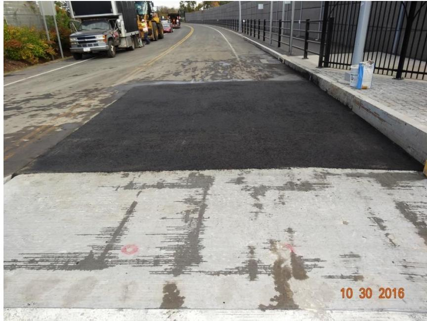
Figure 25. Photo. Completed AC surfacing at the end of the bus pad.
