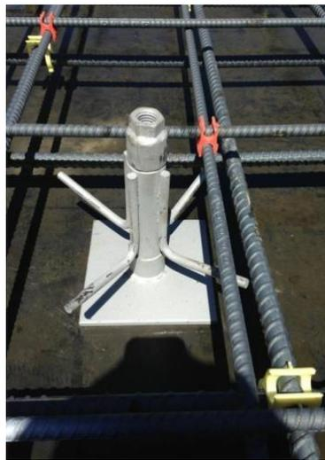
Figure 8. Photo. Gracie leveling lift system.
