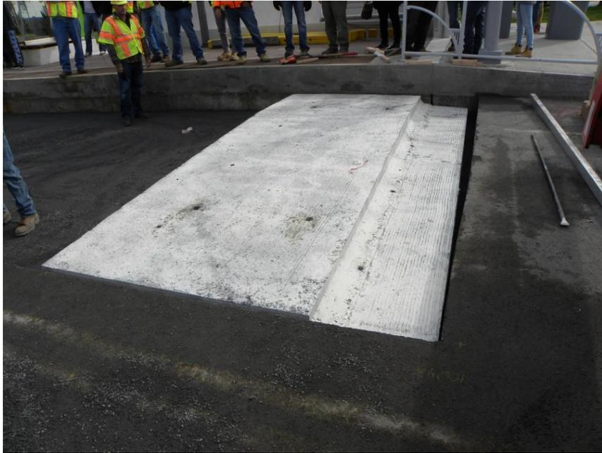
Figure 18. Photo. Misaligned transverse sawcut at the first panel location.
