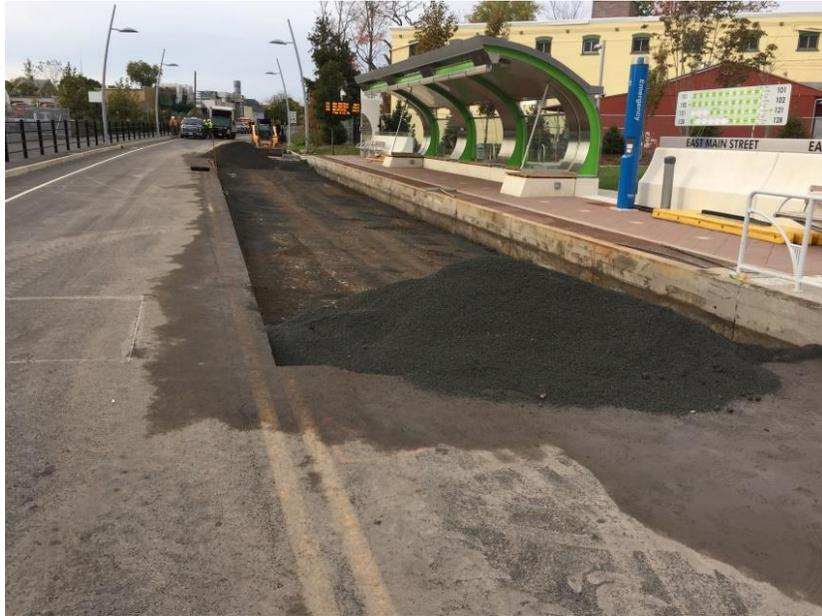
Figure 16. Photo. Removal of the entire bedding layer at the south bus pad.
