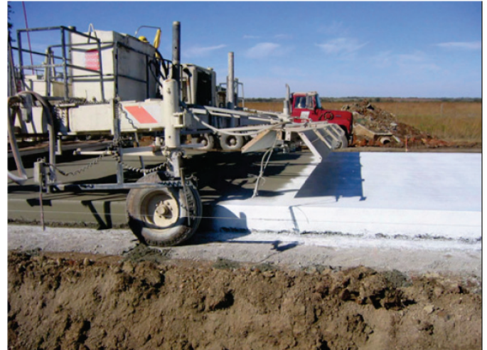
Figure 3. Spray equipment mounted on self-propelled unit applying curing compound to surface and sides of slipformed concrete pavement (Taylor et al. 2007).
