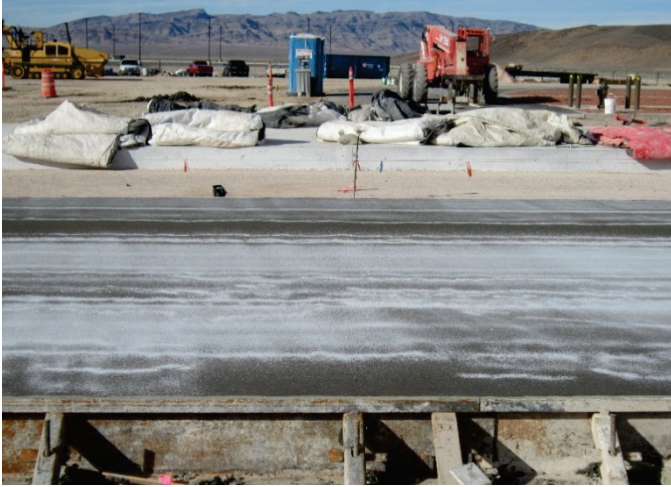
Figure 4. Inadequate application of membrane-forming curing compound.
