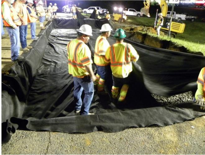
Figure 13. Photo. Geo-fabric placement over the graded and compacted ballast aggregate.
