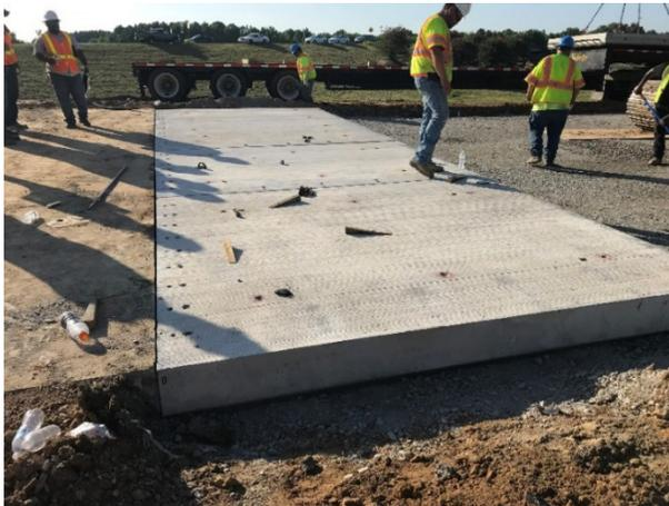
Figure 22. Photo. Stage 3 panel placement – three panels across the roadway width.
