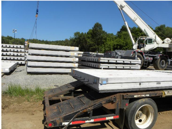
Figure 7. Photo. Staging area for panels.
