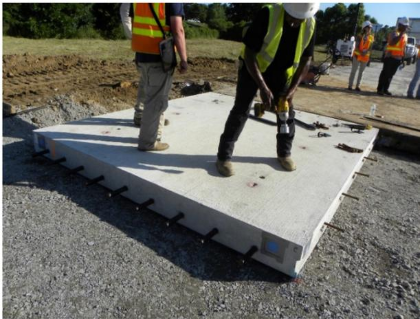
Figure 21. Photo. Use of headed tie-bolts along the longitudinal side of the panel.
