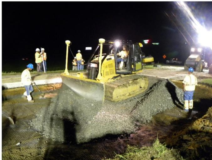
Figure 12. Photo. Ballast aggregate placement.
