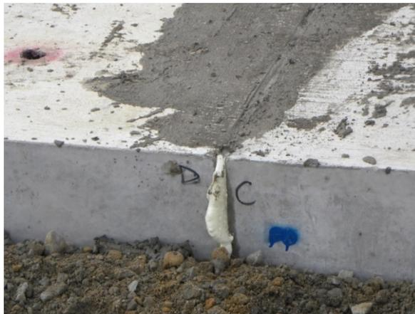
Figure 26. Photo. Polymer foam use at ends of transverse joints to prevent grout leakage.
