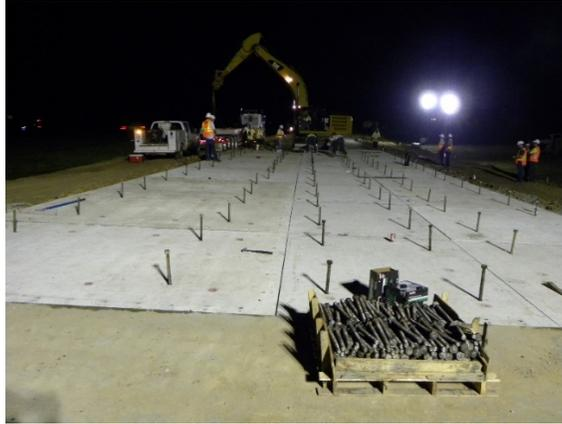
Figure 23. Photo. Stage 3 panels with leveling bolts engaged.
