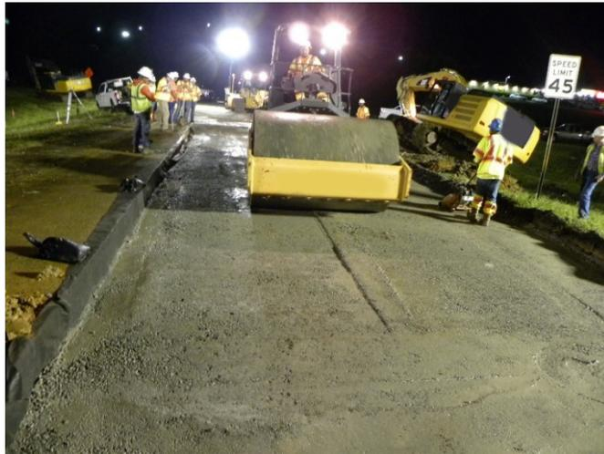
Figure 14. Photo. Base compaction.
