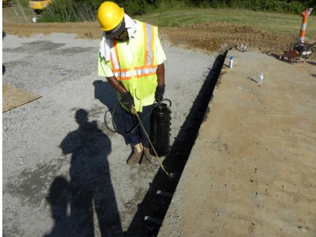
Figure 20. Photo. Debonding liquid being applied to the joint face with embedded dowel bars.
