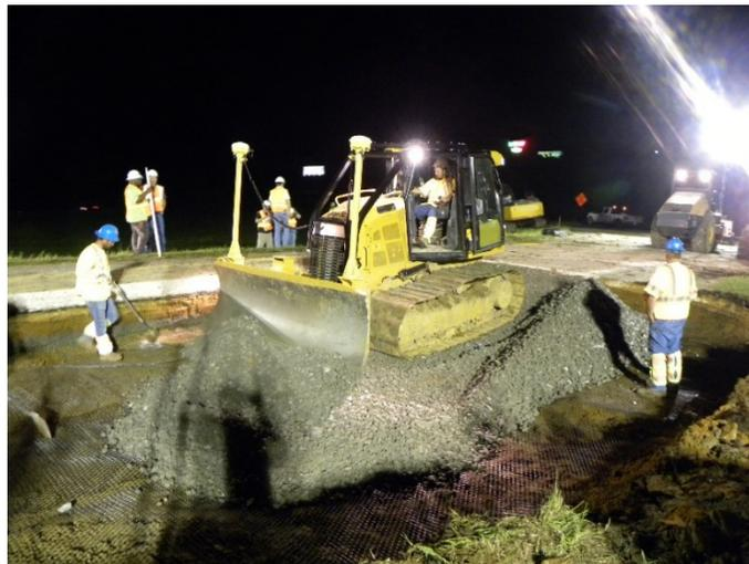
Figure 12. Photo. Ballast aggregate placement.
