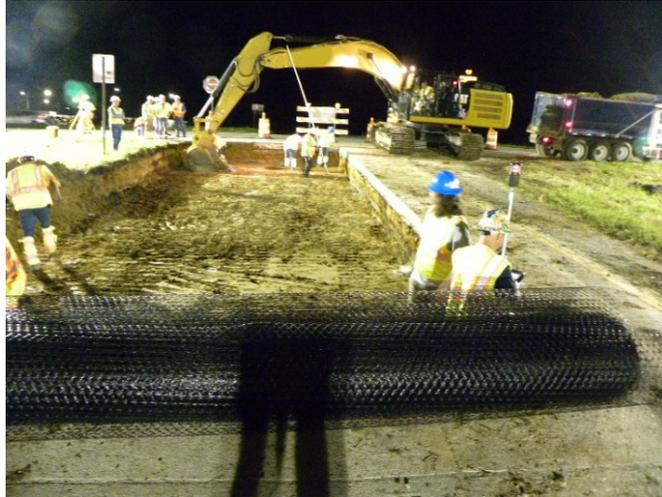
Figure 10. Photo. Subgrade excavation and geogrid for placement over subgrade.
