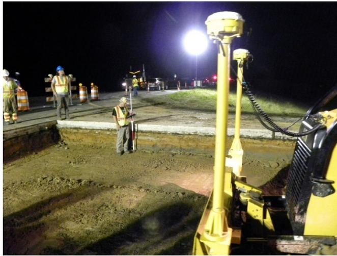
Figure 11. Photo. GPS-based total survey station being used to check subgrade grade.
