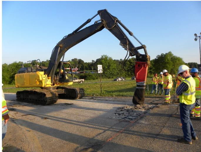
Figure 8. Photo. Existing concrete pavement demolition.
