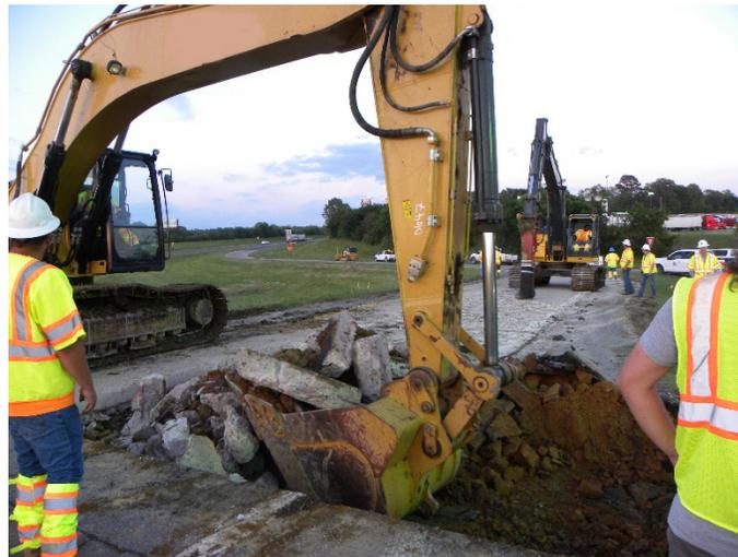
Figure 9. Photo. Broken concrete removal.
