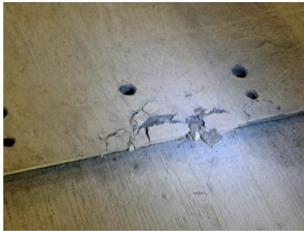
Figure 29. Photo. Stage 3 panel spalling at a transverse joint.
