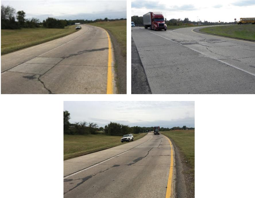
Figure 2. Photos. Cracking in the existing concrete pavement along the ramp.
