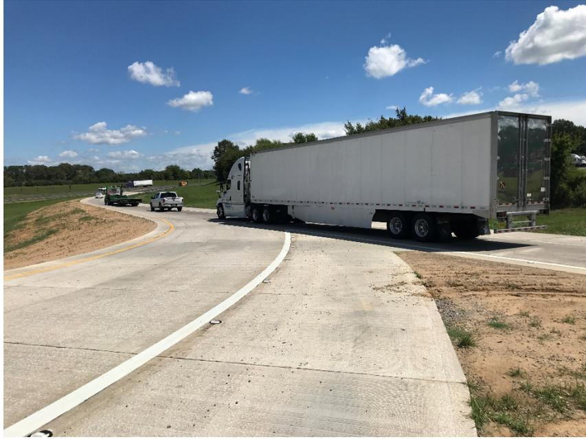
Figure 30. Photo. Completed precast pavement installation.
