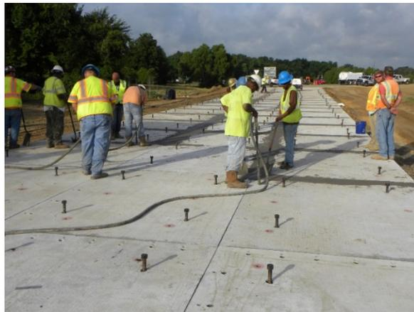
Figure 25. Photo. Stage 3 dowel slot grouting.
