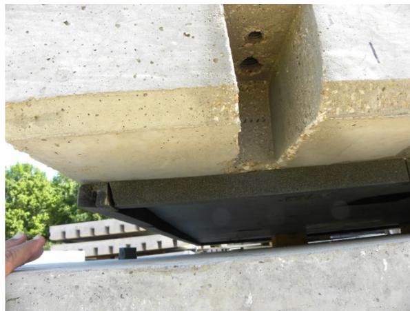
Figure 5. Photo. View of the panel bottom showing gasket around dowel bar slots.
