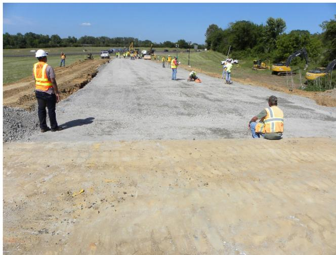
Figure 19. Photo. Base ready for Stage 3 panel placement.
