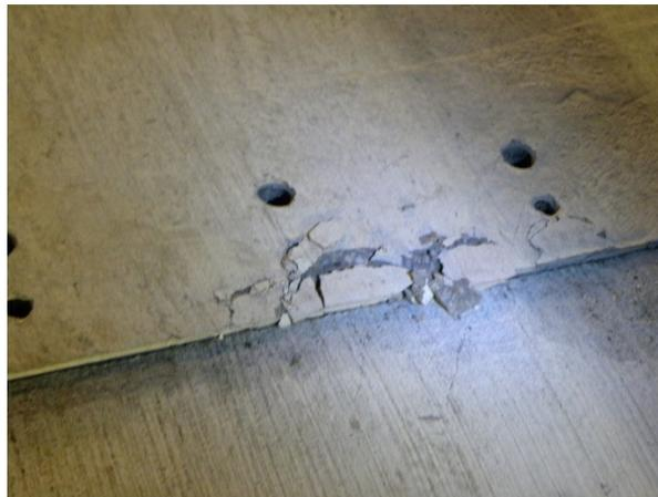
Figure 29. Photo. Stage 3 panel spalling at a transverse joint.
