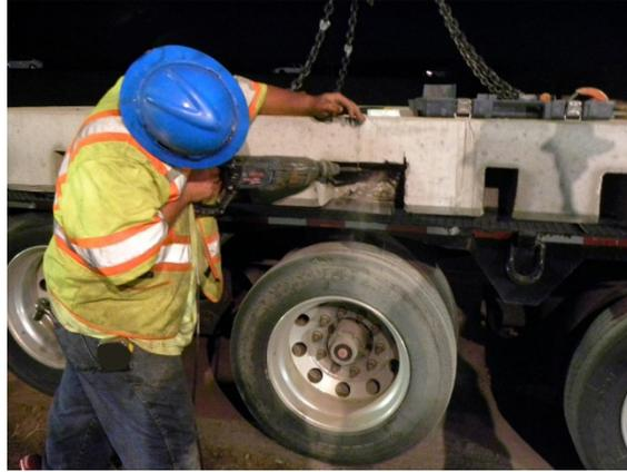
Figure 28. Photo. Panel slot being widened to accommodate mislocated dowel bar.
