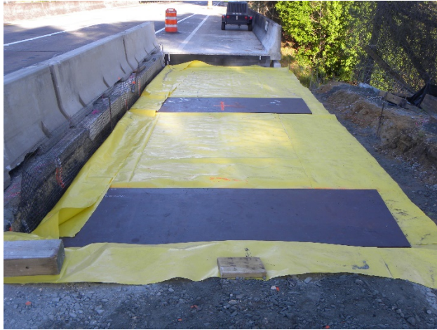
Figure 23. Photo. Bearing plates placed over the polyethylene sheet.
