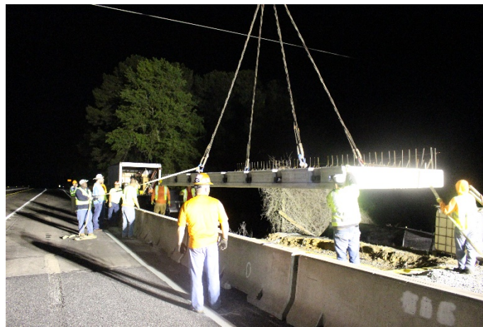
Figure 24. Photo. Panel A being installed.
