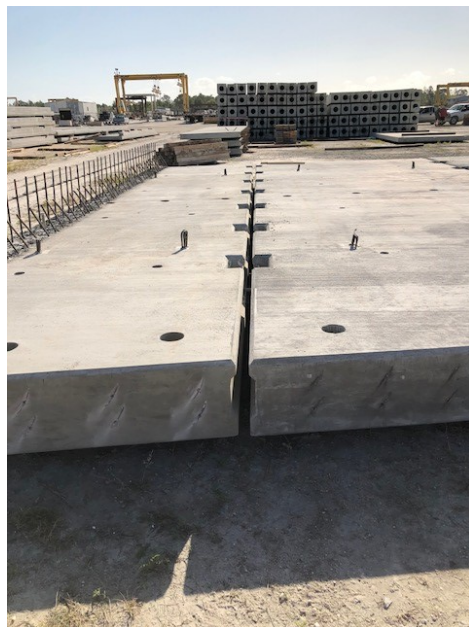
Figure 13. Photo. Longitudinal joint detail.
