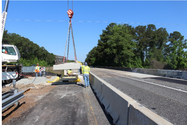
Figure 25. Photo. Panel B being installed.
