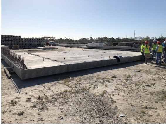
Figure 12. Photo. Mock setup of the four panels at the precast plant.
