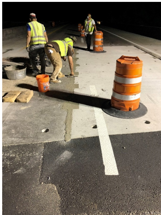
Figure 28. Photo. Longitudinal joint grout installation.
