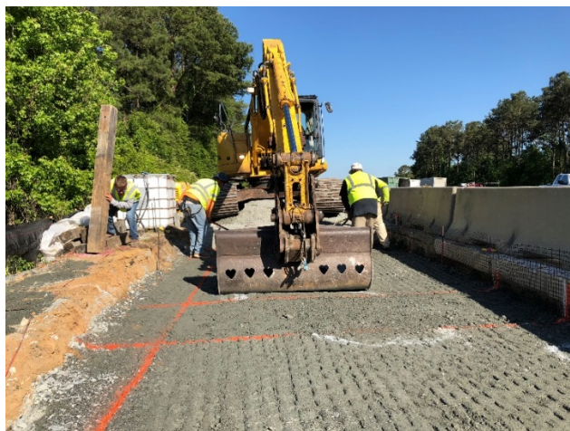
Figure 22. Photo. Base preparation.
