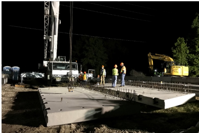
Figure 16. Photo. Panels A and B stored along the median.
