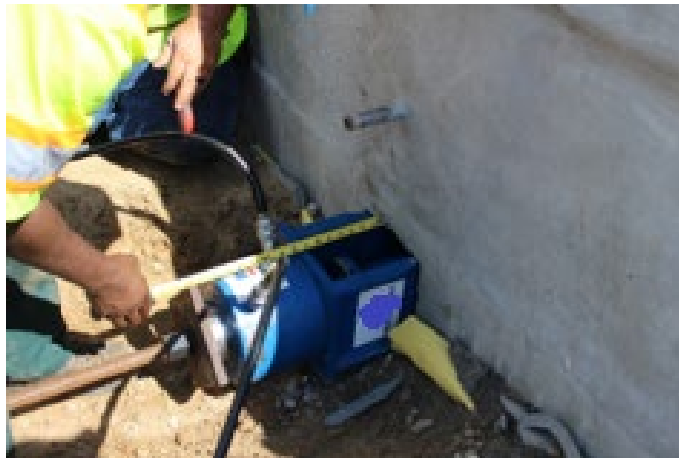
Figure 30. Photo. Posttensioning jack applying load at an anchor plate.
