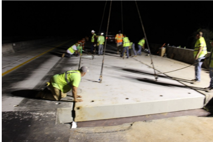
Figure 27. Photo. Panel D being installed.
