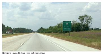
Figure 3. Concrete shoulders using RCA on I-16 in Georgia
