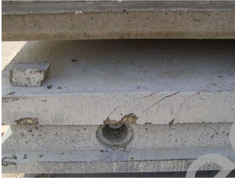
Figure 23. Photo. Damaged panel corner after trial assembly.
