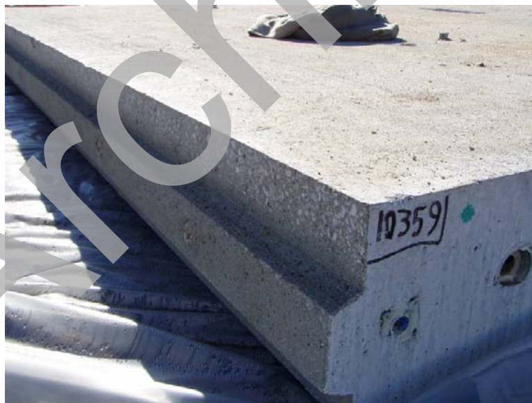
Figure 26. Photo. Keyway after completion of grinding.
