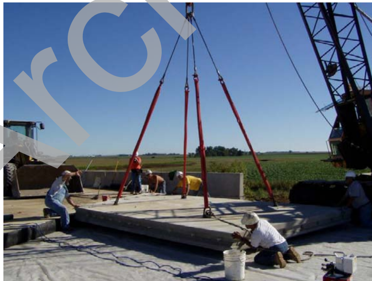
Figure 28. Photo. Installation of Panel 1A at the south bridge abutment.
