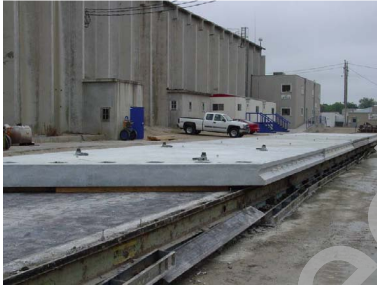
Figure 22. Photo. Trial assembly of precast panels at the fabrication plant (photo by Iowa DOT, reprinted by permission).
