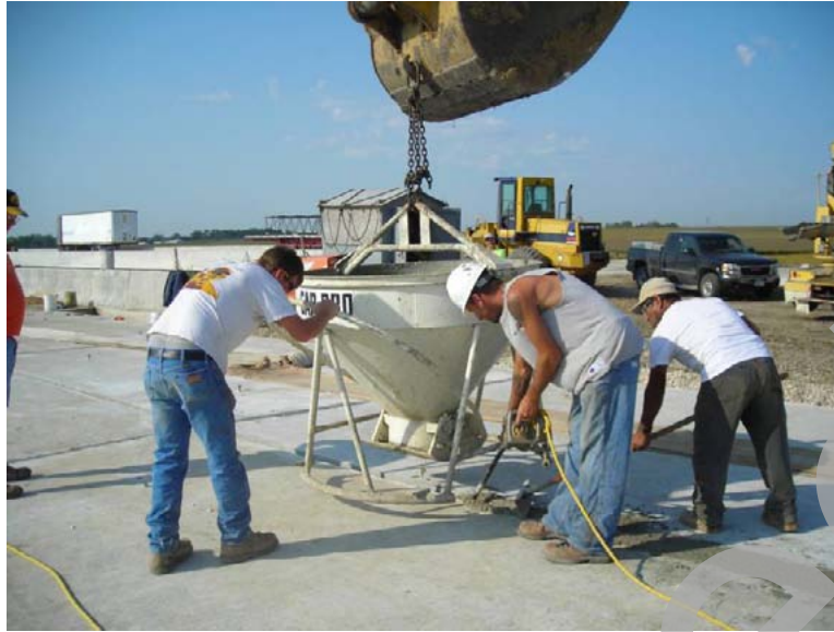
Figure 36. Photo. Filling of the longitudinal joint (photo by Iowa State University, reprinted by permission).
