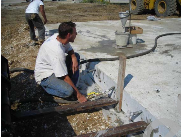
Figure 34. Photo. Grouting of the post-tensioning tendons (photo by Iowa State University, reprinted by permission).
