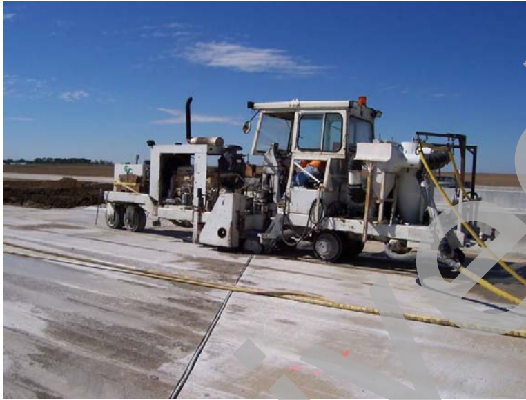
Figure 39. Photo. Diamond grinding the south approach slab.
