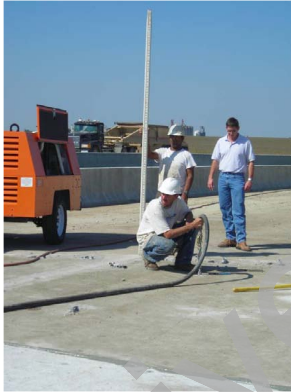
Figure 35. Photo. Rod and level were used to check for slab lifting during the underslab grouting operation. (photo by Iowa State University, reprinted by permission).
