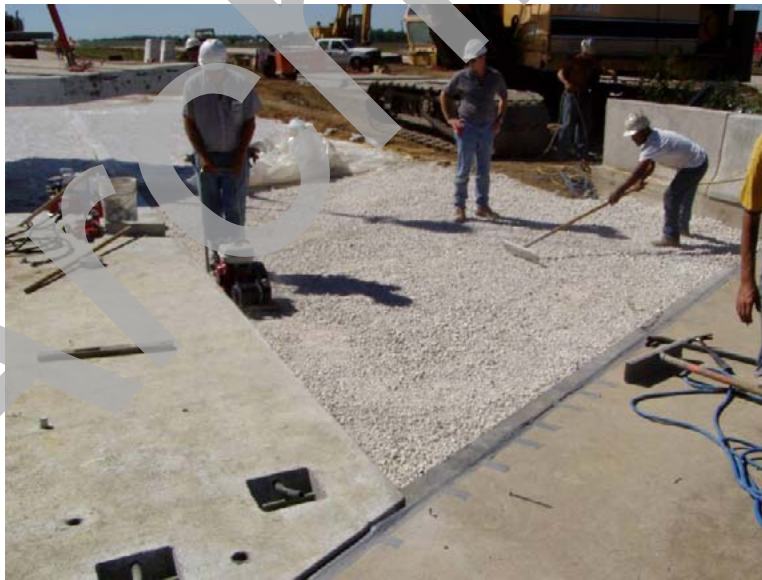
Figure 27. Photo. Grading and compaction of the aggregate base material.
