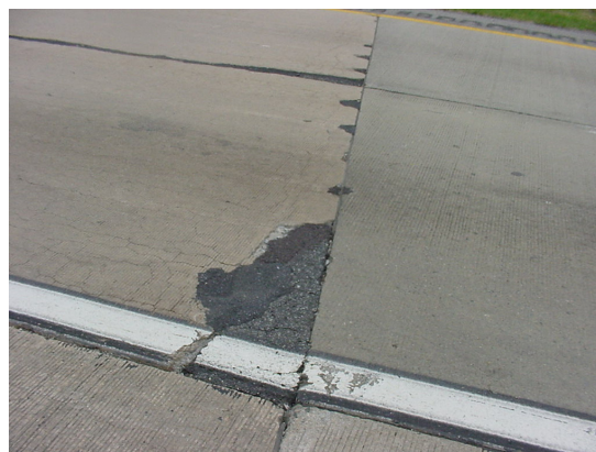
The left side of the image shows the section of SR-1 that had no ASR mitigation and was overlaid with NovaChip and a 2-inch hot mix asphalt layer. The right side of the pavement was constructed with slag cement as an ASR preventative effort.
