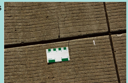
Cracking seen on US 113 near Georgetown, Delaware.
