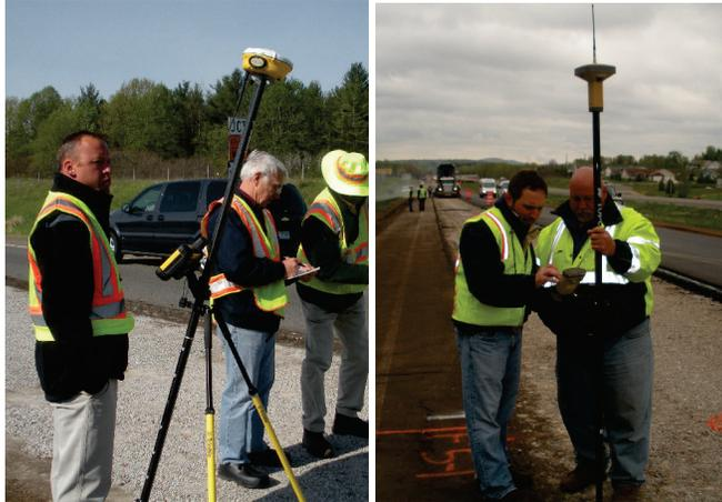
**Figure 193. A Trimble GPS rover (left) and a TopCon GPS rover (ICPF WisDOT demo).**
