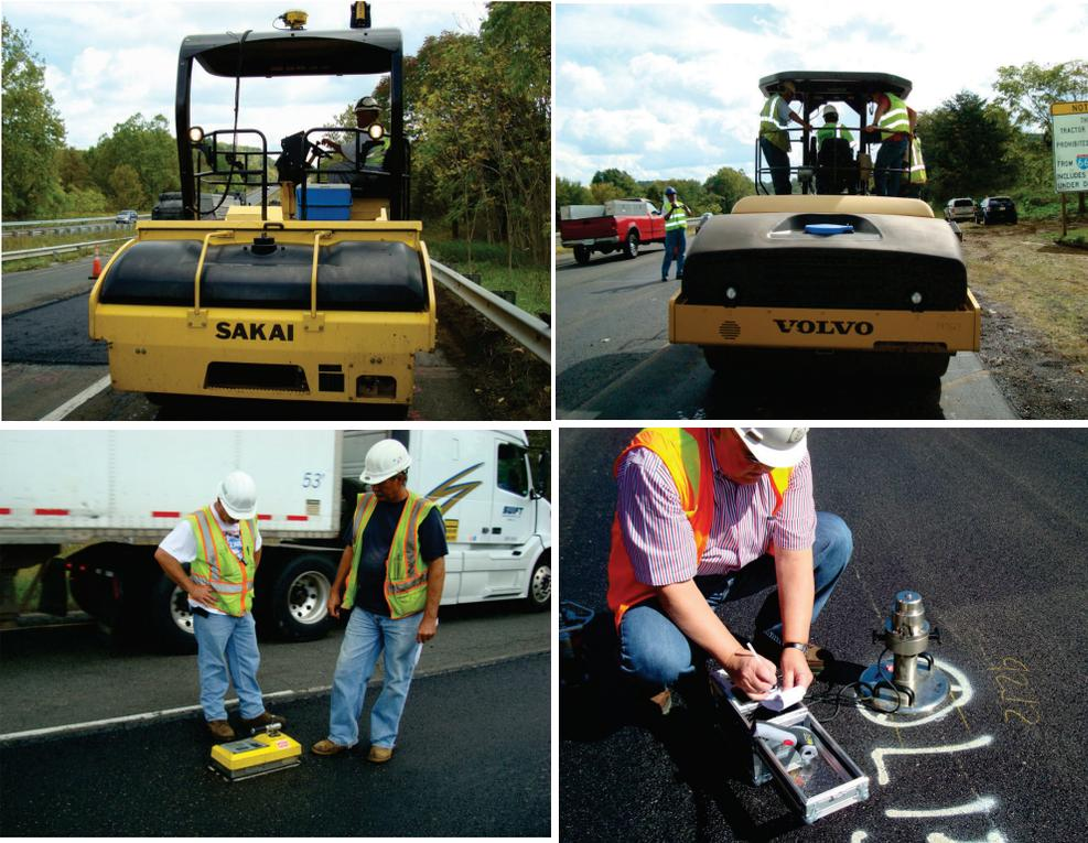
Figure 158. Virginia HMA IC demonstration.
