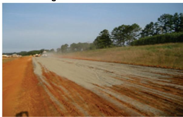
**Placement of cement on moist-conditioned subgrade**
