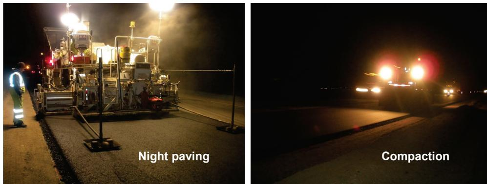
**Figure 145. Night paving and HMA compaction.**
