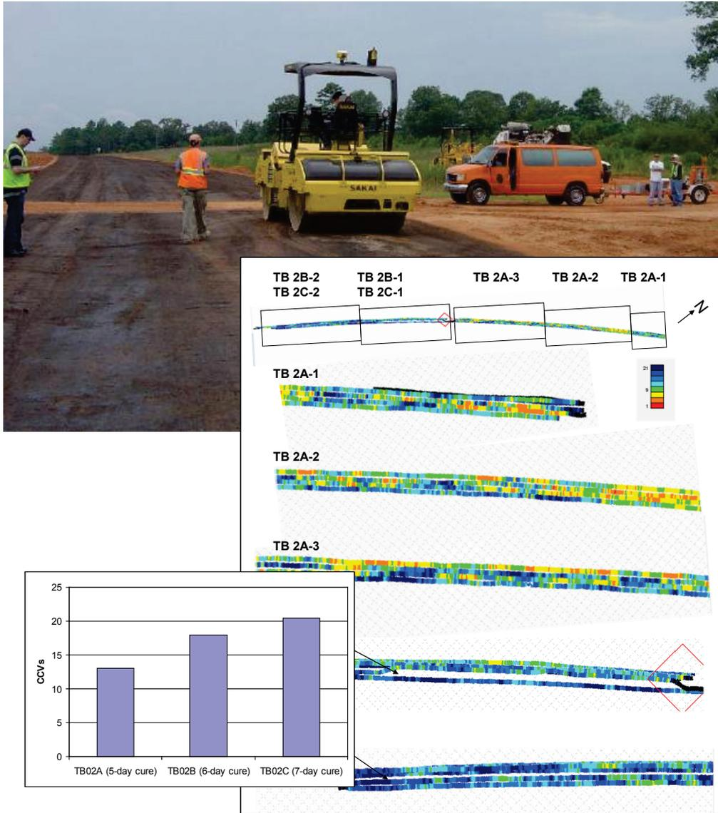
**Figure 107. Mapping of tack-coated, stabilized subbase with the Sakai double-drum IC roller.**
