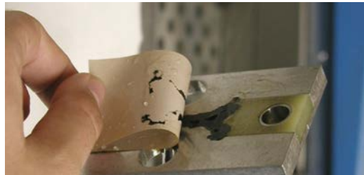
Figure 54: Removing release paper
