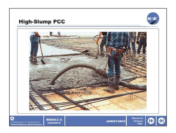
The high-slump PCC shown in this photo is common for pump delivery for flatwork and form placement. A major advantage of using a high range WRA or superplasticizer is that the segregation potential of the mix is minimized. Segregation is oftentimes a result of over-vibration so when the mix is sufficiently fluid to minimize the need for vibration, the segregation potential decreases.
