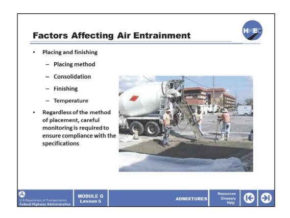
Placing, whether hand placement, machine placement, or pumping tends to reduce the entrained air content by varying degrees depending on the mix characteristics. Hand placement typically uses a relatively high slump mix that can lose air relatively easy if overvibrated during consolidation.
