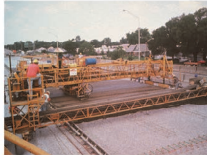
Placement, strike off, consolidation, and finishing using fixed form techniques
