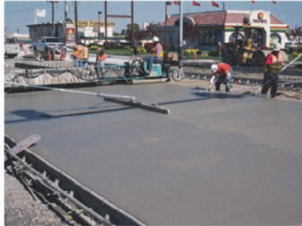
Typical urban fixed form paving operation
