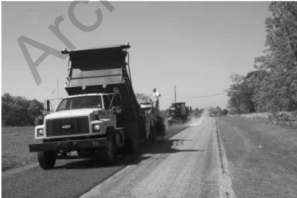
State and local highway agencies are applying more and more preservation treatments to their roads, such as the chip seal shown here.
