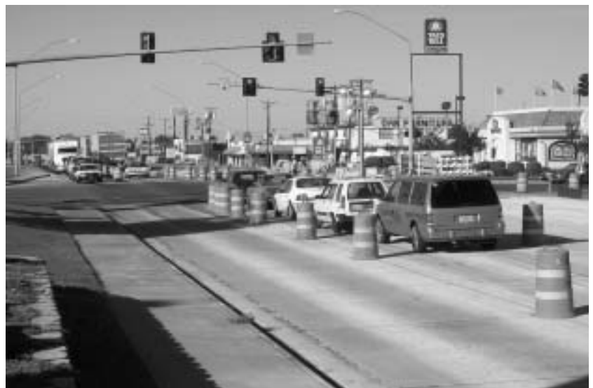
Three intersections in Kennewick, Washington, were completely closed to traffic for 3 days, allowing for uninterrupted reconstruction work.
