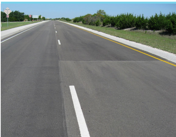
Advanced, proven preservation practices can help extend the overall service life of pavements.
