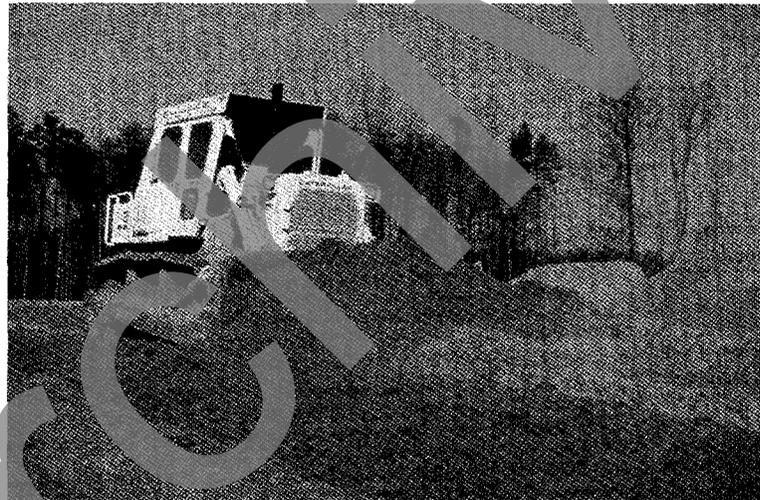
Figure 22. Spreading fly ash structural fill.
