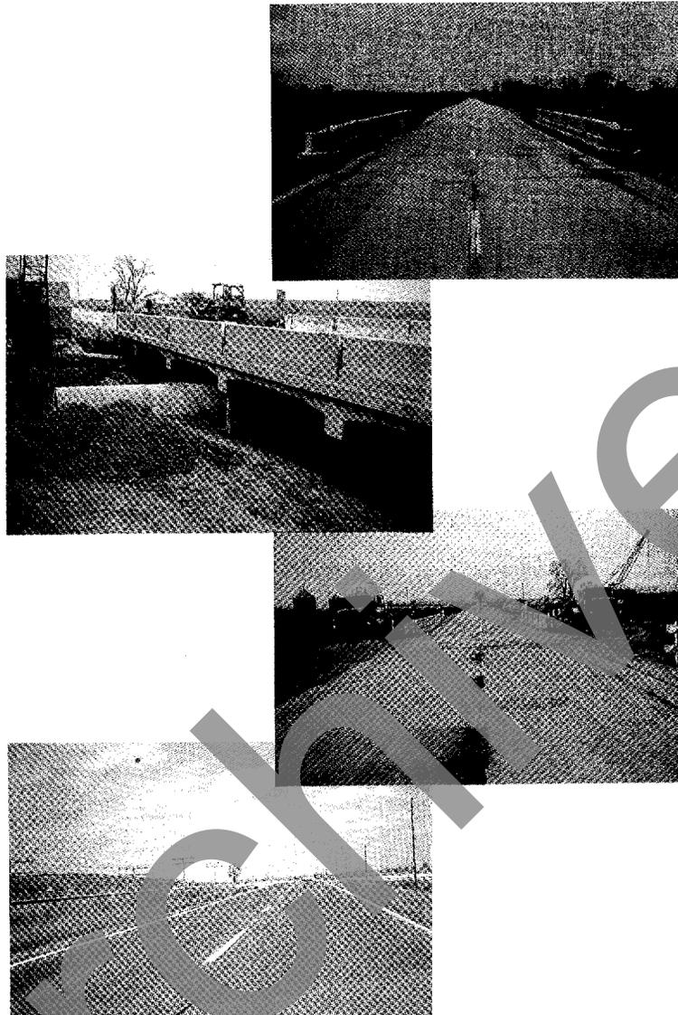
Figure 18. Bridge replaced by culverts and flowable fill.
