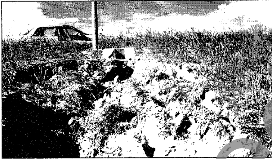
Photo No. 10 Outlet Erosion
