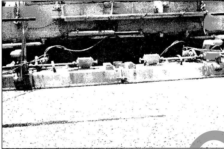
Photo No. 8. Compacting Cement Stabilized Permeable Base Material
