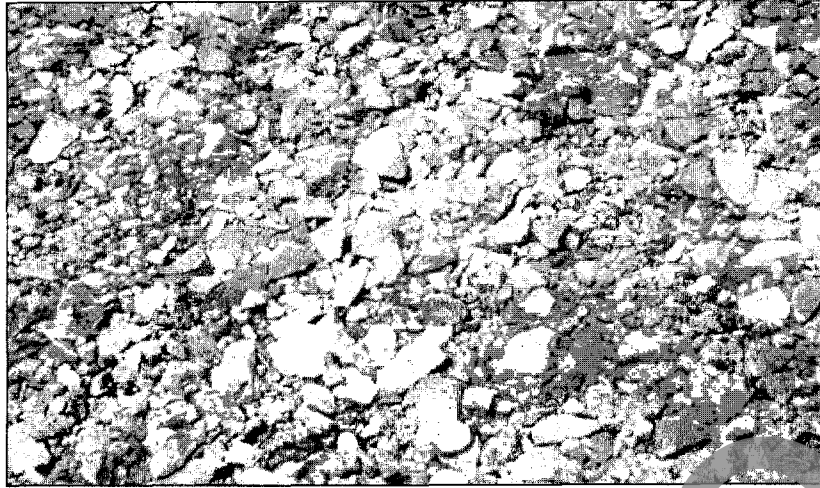
Photo No 4. Completed Unstabilized Permeable Base
