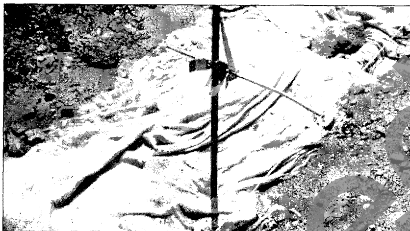
Photo No. 3 String Control for line and Grade
