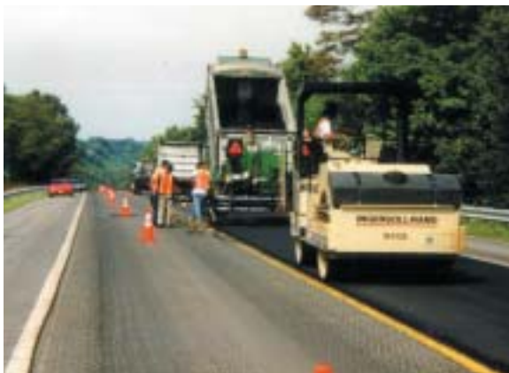
Figure 17. Construction of HMA pavement
