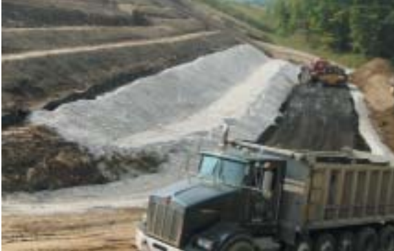
Figure 9. Foundry sand delivery (sand supplied by Kurtz Bros., Inc., construction by Trumbull Corp.)
