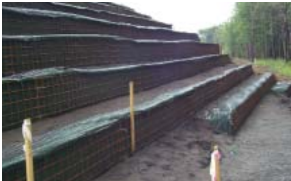
Figure 12. Stepped embankment (Ohio turnpike, sand supplied by Kurtz Bros. Inc., construction by Trumbull Corp.)
