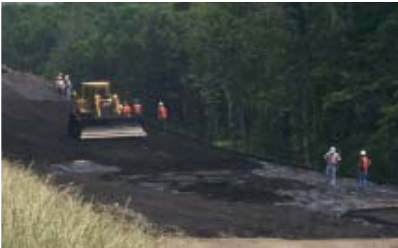
Figure 10. Spreading foundry sand (Ohio turnpike, sand supplied by Kurtz Bros. Inc.)
