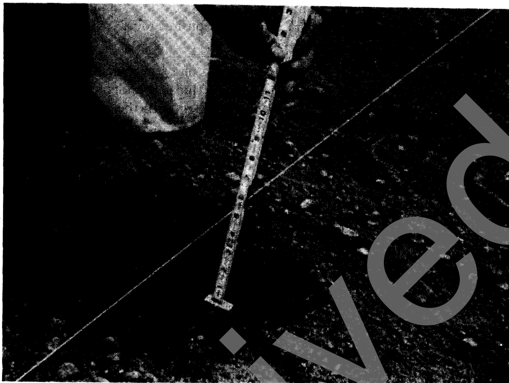
FIGURE 5.6—Grade and Line Stakes.
