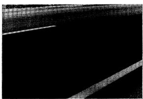
Reviews in several States indicate that micro-surfacing placed over thermoplastic material will ravel off the marking. Accordingly, thermoplastic and cold plastic marking (and preferably paint marking) should be scarified or removed prior to micro-surfacing application.
