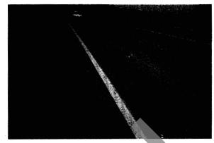
Micro-surfacing has been used to repair OGFCs and raveled surfaces with considerable sucess. This slide shows a 3 years old micro-surfacing project placed on top of a raveled OGFC project in Oklahoma
