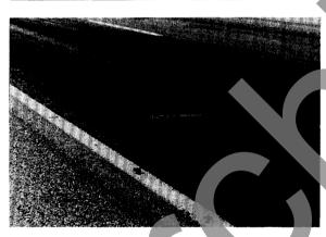
Micro-surfacing has been used by some States to correct/minimize flushing on chip seals and asphalt concrete pavements. Micro-surfacing use on flushed pavements should be limited to sites where flushing is low to moderate, otherwise flushing may reappear.
