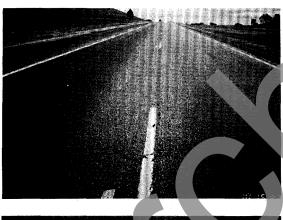
This is a 5-years-old micro-surfacing project on I-40 in Oklahoma. This project involved both rut filling and texturing. With the exception of minor wheel consolidation and cracking, the surface is in good condition.
