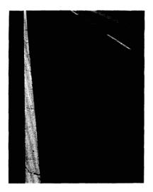
This slide shows a drag mark caused by sealant build up on the surface.
