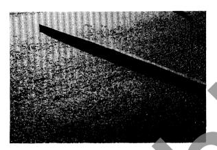
Several States have experienced instances of bleeding when filling ruts of 40 mm or more in a single pass. The coarser aggregate fraction can settle into the deeper rut areas, leaving binder-rich fines at the surface and resulting in a low or uneven surface texture and the unsightly appearance of "fatty spots."
