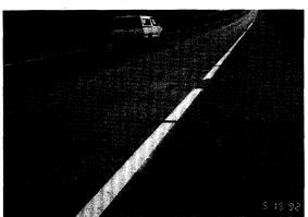
This is a three years old rut filling project on I-94 in Wisconsin. While some "shadow" spots are visible, the project did not exhibit reformation of significant ruts (i.e., ruts in excess of 12.5 mm rerutted to only 5mm).
