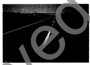
This slide shows a micro-surfacing project 30 to 45 minutes after application. This contrast in texture is usually caused by a wet mixture.
