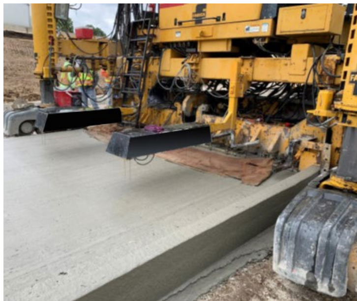
LEFT: Engineer Eric Desjardins uses the Instant Air Meter during a cooperative agreement demonstration event. RIGHT: Non-contact sensors measure real-time smoothness of freshly paved concrete during a demonstration. (Source: Concrete Pavement Technology Center)
