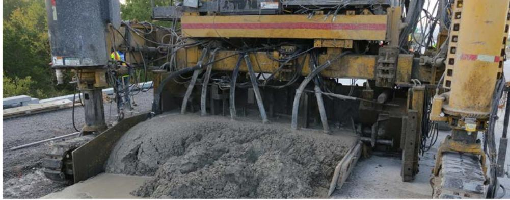
*Two-lift concrete paving, as shown here, uses a higher percentage of recycled or marginal aggregate in a thicker bottom layer, while reserving more durable material for the thinner surface layer, thereby improving the sustainability of the pavement without compromising performance. Source: APTech.*
