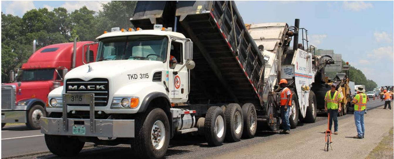
Crews in Florida are constructing experimental sections as part of a demonstration project to evaluate the performance of asphalt pavements with increased compaction density. Source: NCAT.
