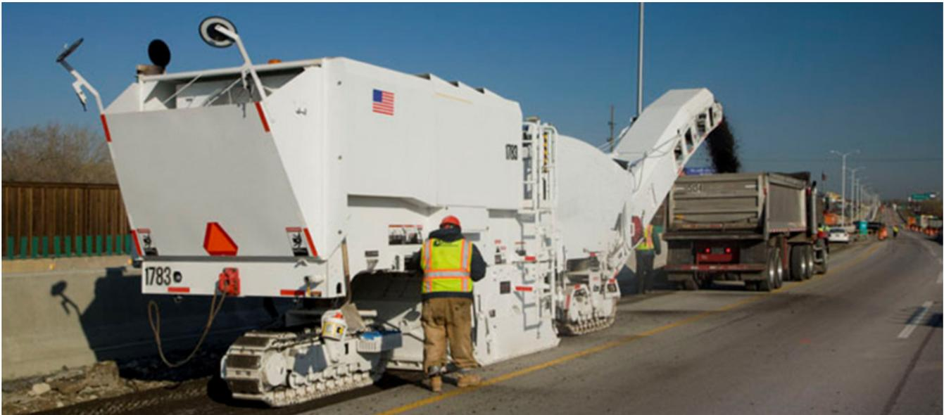
A milling machine is removing layers of asphalt pavement to generate recycled asphalt pavement, or RAP, as part of a rehabilitation project.
