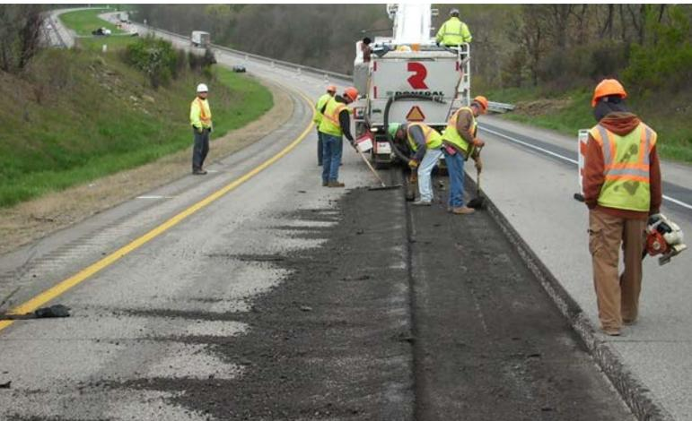
A crew is repairing a longitudinal joint in Pennsylvania using a mill and fill patching process along the full length of the pavement.
