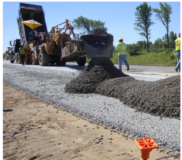
Figure 2. Concrete placement through the use of a belt conveyor.
