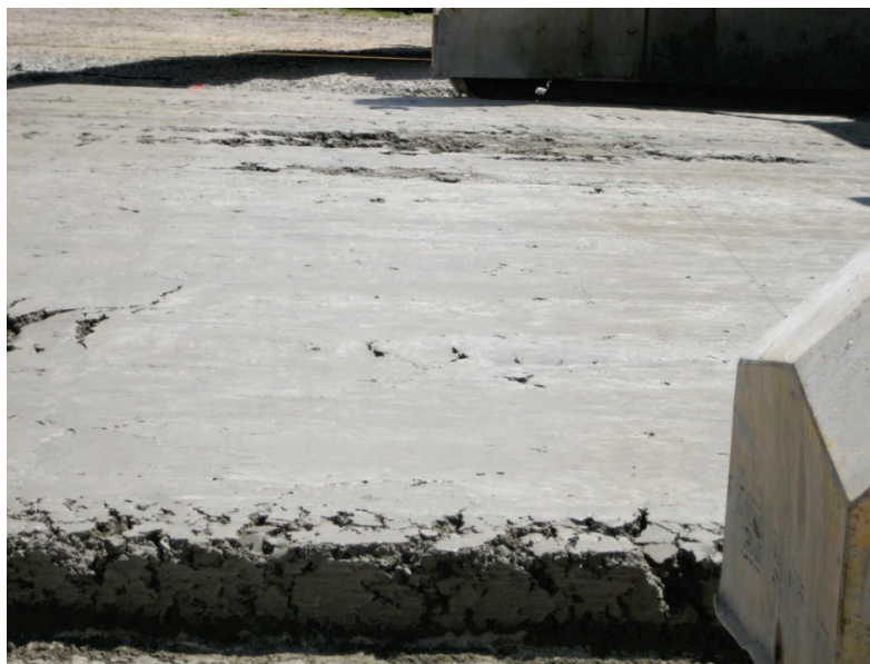
Figure 28. Tearing of top-lift concrete surface caused by dried concrete on profile plan.
