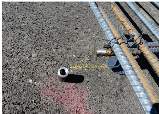
Figure 35. Threaded coupler used in two-piece tie bar system.
