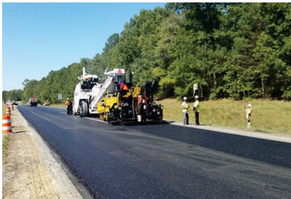
Figure 20. Paving of the SMA in the driving lane of the Virginia HMA/CRCP project.
