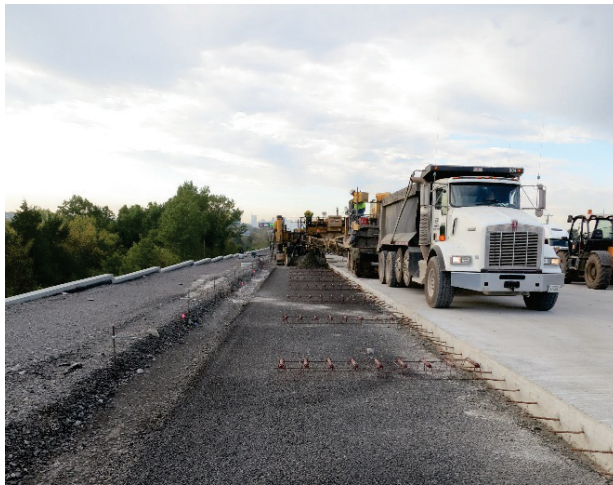
Figure 27. Tennessee PCC/PCC composite pavement project: bottom-lift material delivered by end-dump truck (left photo) and top-lift material delivered by a front-discharge ready-mix truck (right photo).
