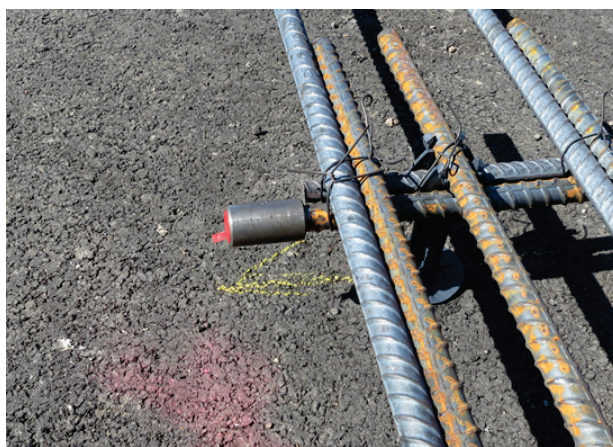
Figure 35. Threaded coupler used in two-piece tie bar system.
