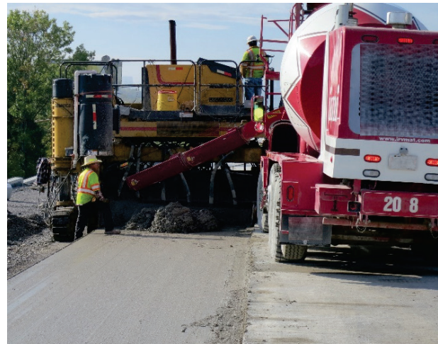
Figure 27. Tennessee PCC/PCC composite pavement project: bottom-lift material delivered by end-dump truck (left photo) and top-lift material delivered by a front-discharge ready-mix truck (right photo).
