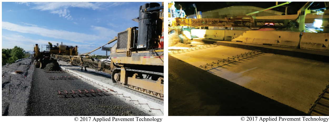
Figure 22. Dowel baskets on grade on two-lift paving projects in Tennessee (left photo) and California (right photo).
