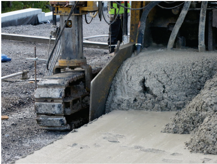
Figure 32. Crowning of bottom lift with top lift material on Tennessee PCC/PCC project.
