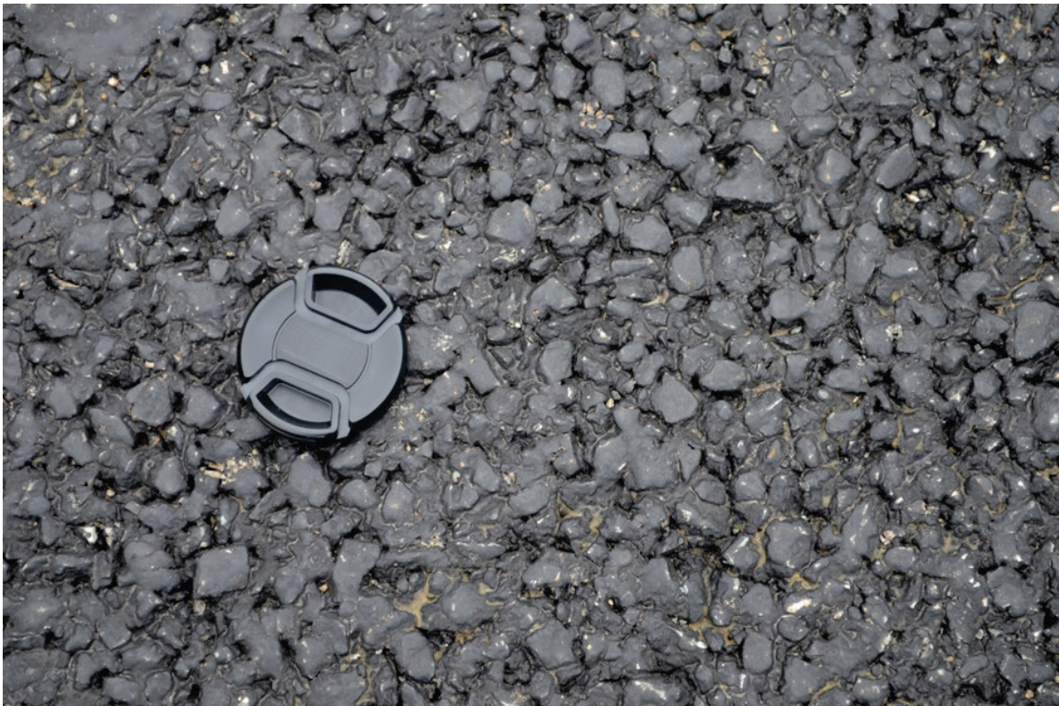
Figure 13. Close-up of stone matrix asphalt (SMA) surface (Ram and Smith 2018).
