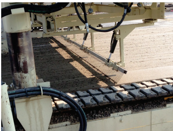
Figure 37. Longitudinal (left, Illinois Tollway) and transverse (right, Tennessee I-65) tining on PCC/PCC composite pavement projects.
