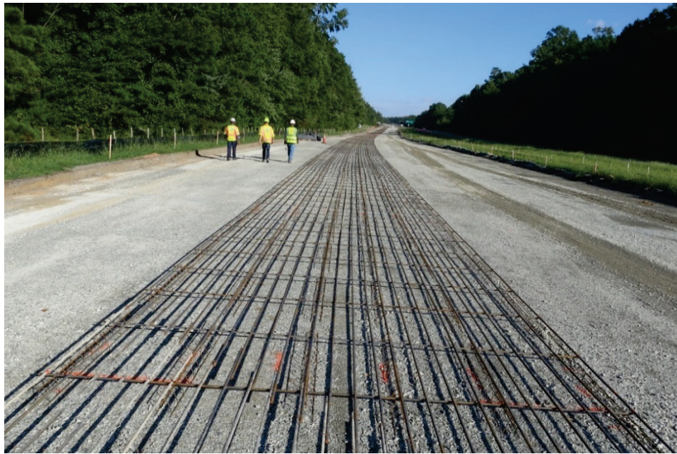
Figure 18. Reinforcing steel layout for one lane of Virginia HMA/CRCP composite pavement.
