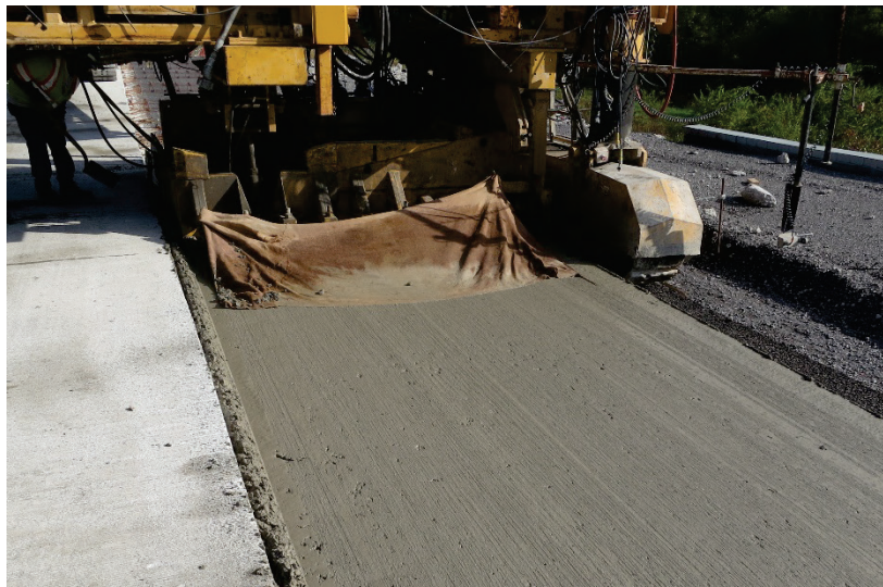
Figure 29. Drag texturing of bottom lift on Tennessee PCC/PCC project.
