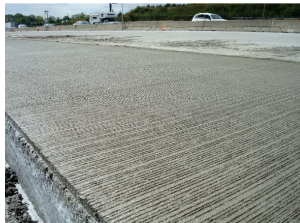
Figure 37. Longitudinal (left, Illinois Tollway) and transverse (right, Tennessee I-65) tining on PCC/PCC composite pavement projects.
