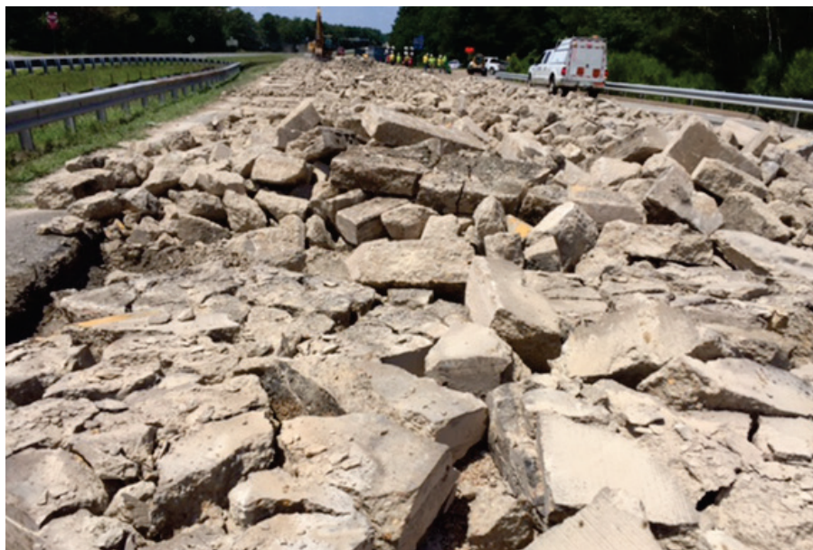
Figure 17. Broken up CRCP pavement on grade.
