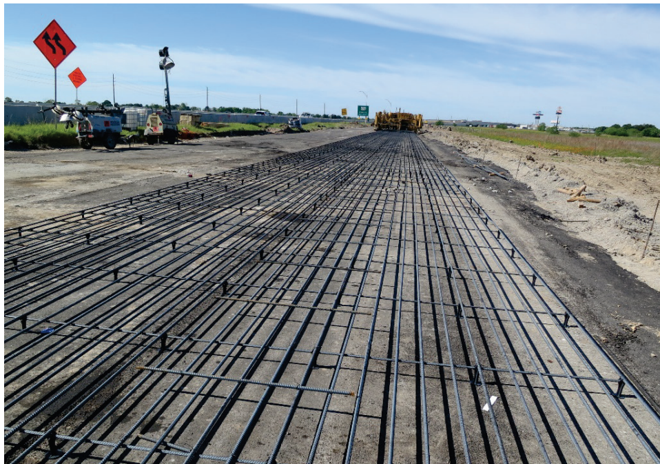
Figure 25. Layout of reinforcing steel for outside lane and outside shoulder of Texas PCC/PCC composite pavement.
