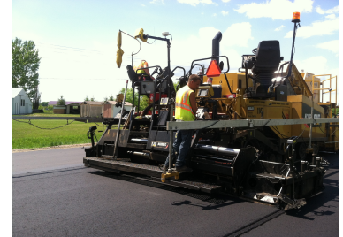
Above: A PMTP in use on a paver in Minnesota. Photo: MnDOT. Below: Sample of a thermal map. Image provided by FHWA.
