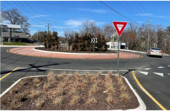
Figure 6. Completed PCP truck apron of roundabout.
