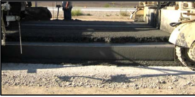
Figure 5. Two-lift concrete paving (image credit: Peter Taylor).
