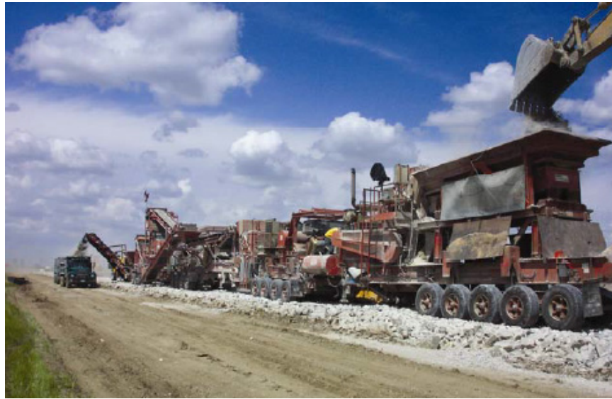
Figure 8-9. Recycling existing concrete pavement in place (photo courtesy of Jim Grove).
