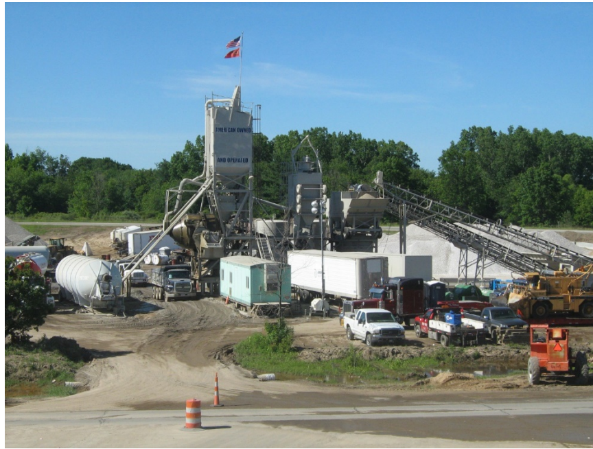
Figure 8-8. On-site concrete recycling operation.
