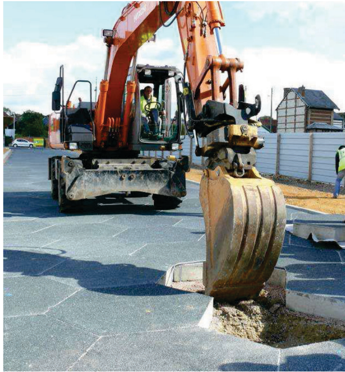
Figure 9-9. Removal of French hexagonal modular pavement to access utility (Larrard, Sedran, and Balay 2012).
