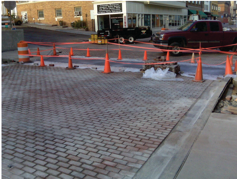
Figure 9-3. Vehicular interlocking concrete pavers being placed in a pedestrian-friendly downtown area in Houghton, MI. Note the use of colored concrete for the pavers to provide a visual offset for the cross walk (photo courtesy of Thomas Van Dam).
