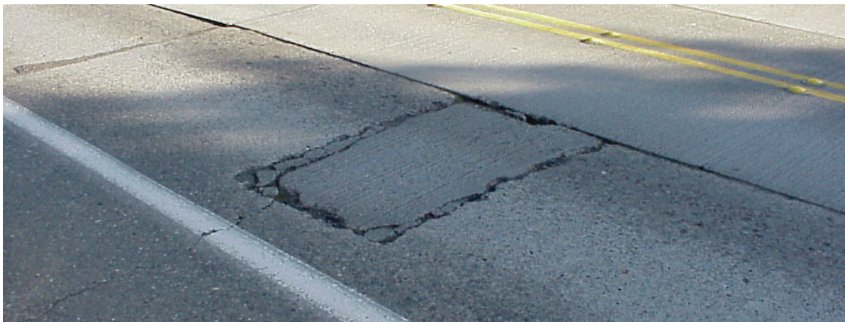
Figure 9-7. Poor quality patch in an existing concrete pavement (photo courtesy of Steve Muench).
