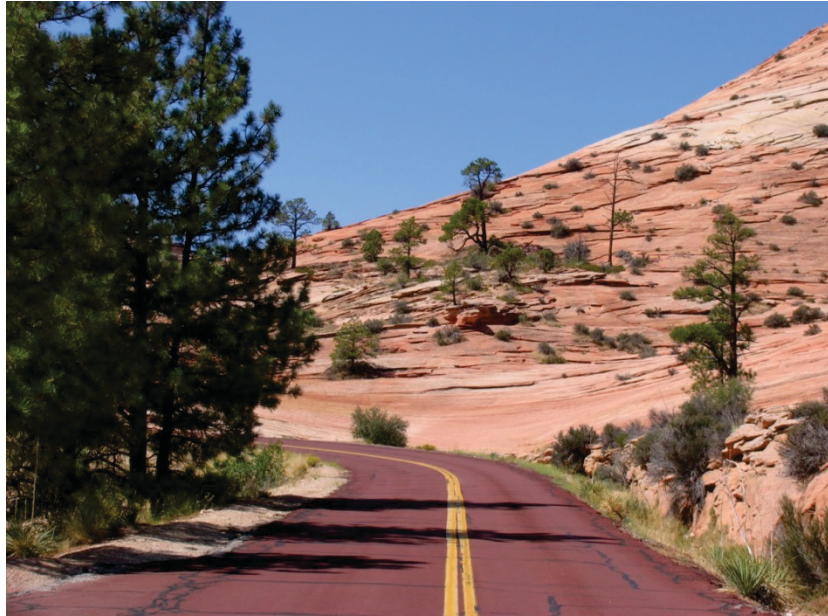
Figure 9-1. Zion Park Blvd. in Utah (SR 9) with a chip seal surfacing that uses local red volcanic cinders to match the aesthetics of the surrounding environment and to be consistent with historical road surfacing (photo courtesy of Steve Muench).
