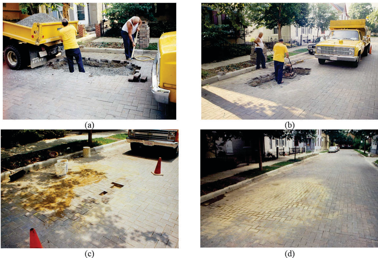
Figure 9-8. Illustration of how existing concrete pavers can be removed to repair a gas line (a), and then the bedding recompact (b), joint sand reapplied (c), and the final product which shows little sign of disturbance (d) (ICPI 2009).
