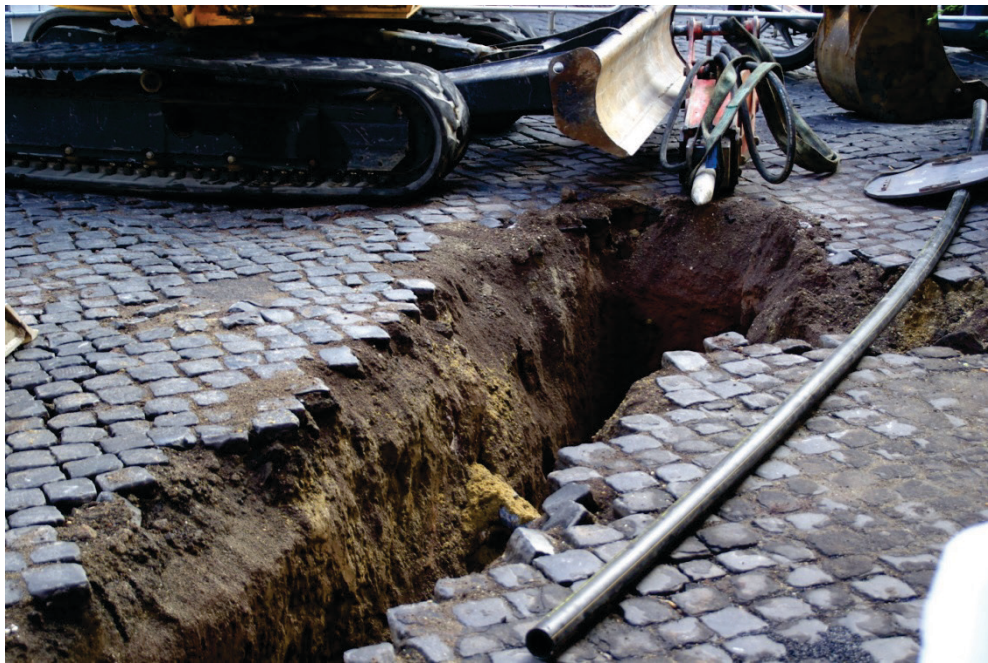
Figure 9-10. A utility cut in Rome, Italy shown with the excavation open and sampietrini (individual rounded black basalt stones) removed. Upon completion the cut is filled and sampietrini reinstalled (photo courtesy of Steve Muench).
