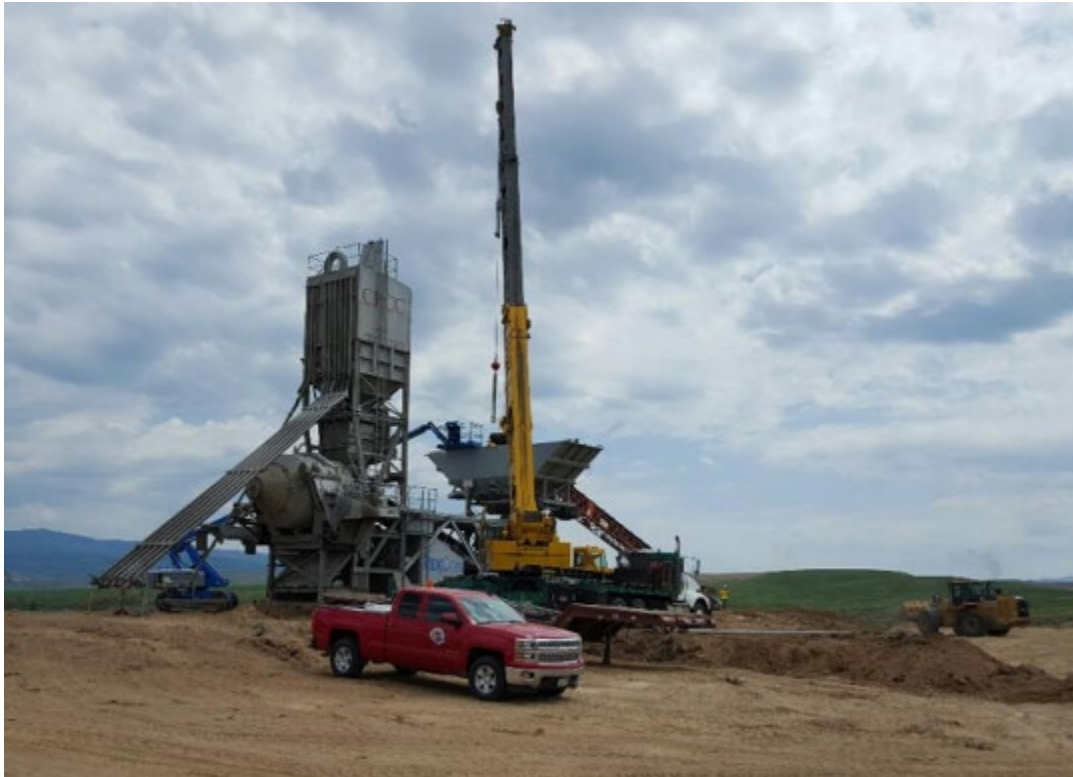
Photo: Castle Rock Construction Company, used with permission
