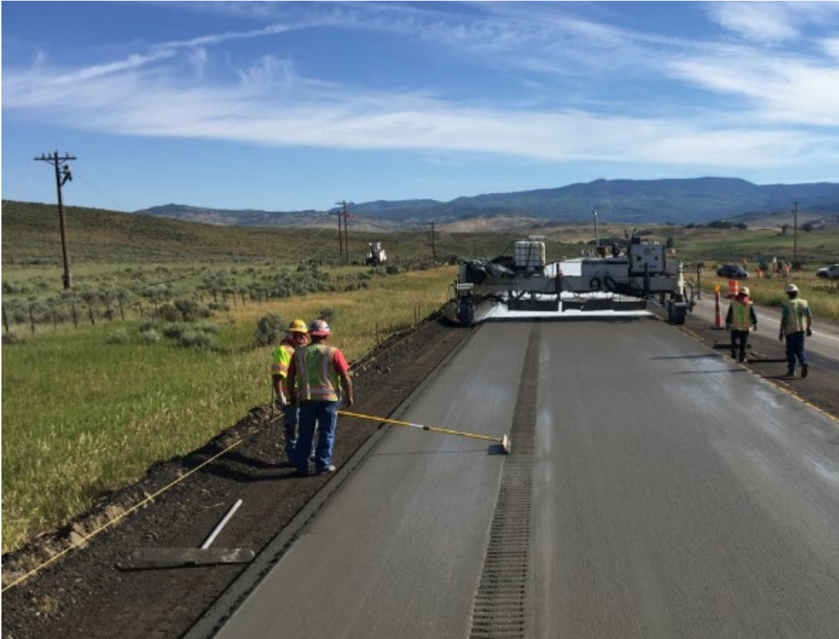
Photo: Castle Rock Construction Company, used with permission
