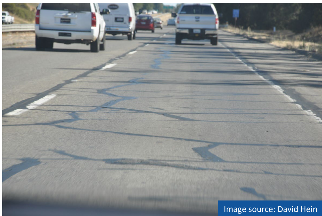
HMA or WMA Pavement
