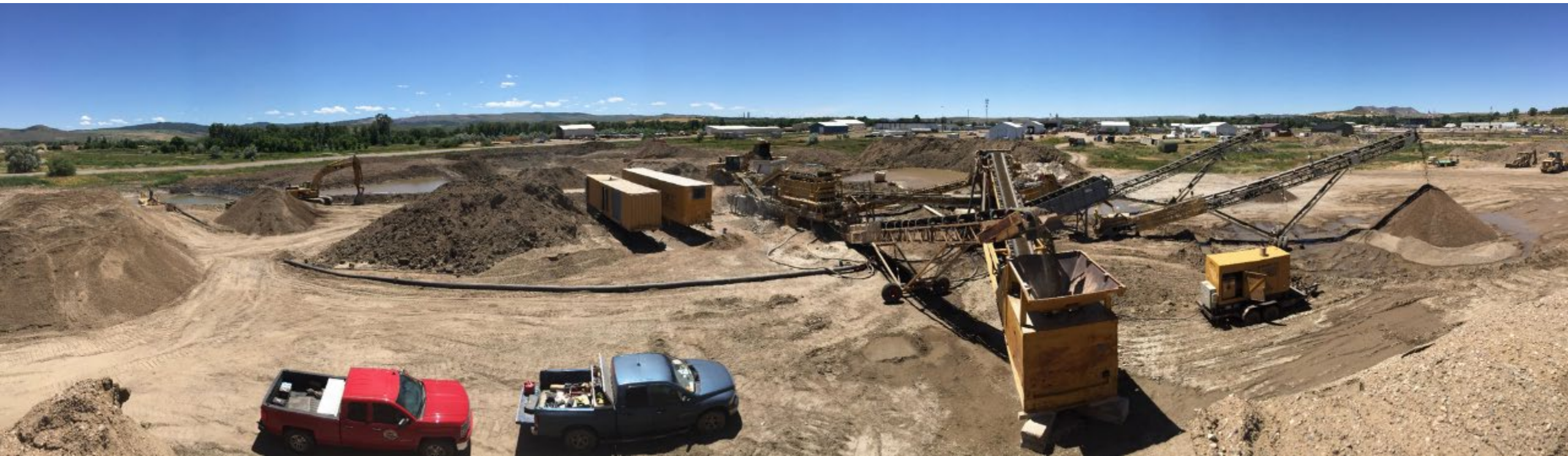
Photo: Castle Rock Construction Company, used with permission
