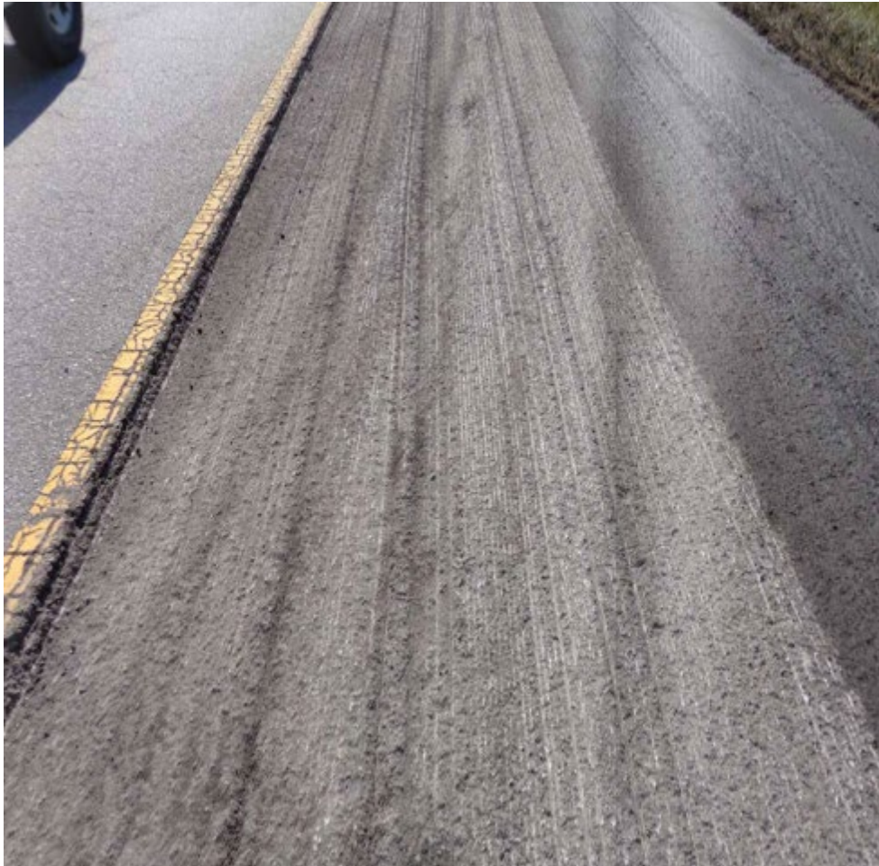
Photo: Castle Rock Construction Company, used with permission
