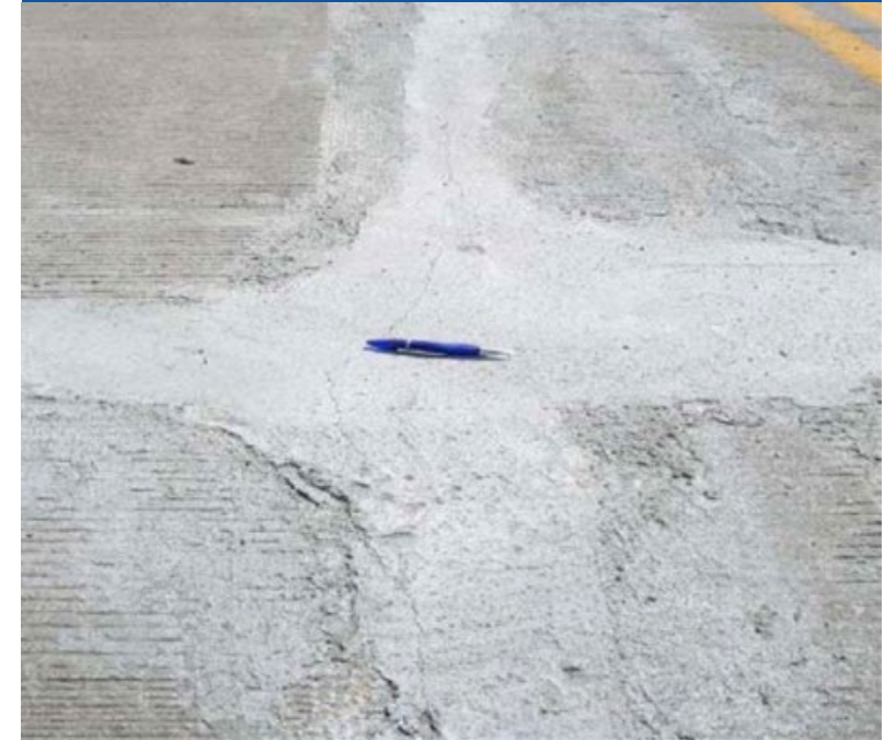
Spalls Filled with Flowable Mortar
