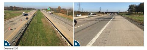
Figure 1. Concrete overlay on I-495 in Delaware in 2020: (a) going northbound and southbound and (b) close-up view of the overlay
