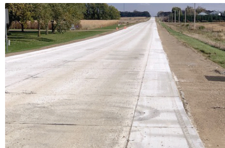
Figure 3. Completed overlay
