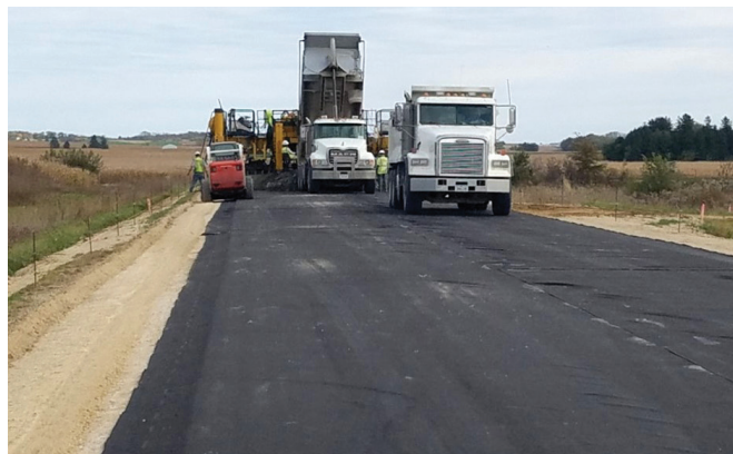
Figure 2. Placement of a concrete overlay on a nonwoven geotextile separation layer
