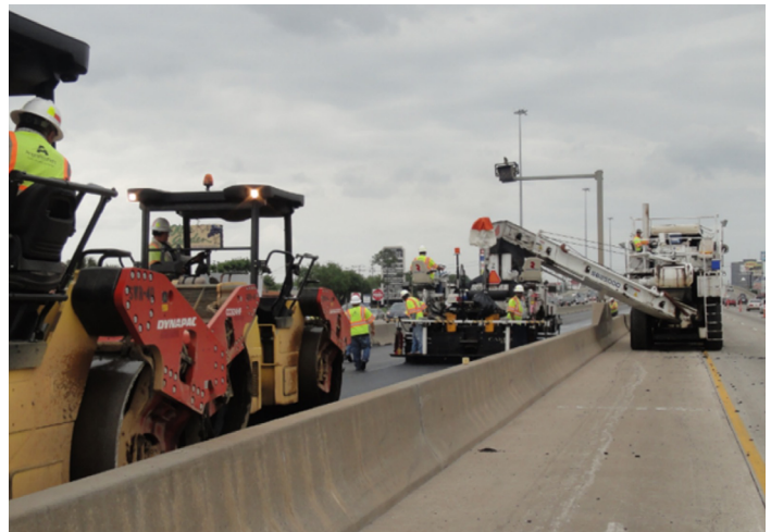
Construction of the Interstate 69 overlay system.
