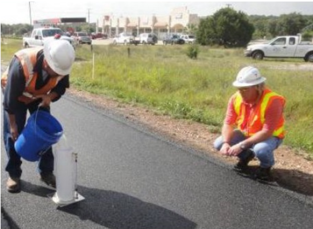
Figure 17. Water flow test. Source: TxDOT Austin District
