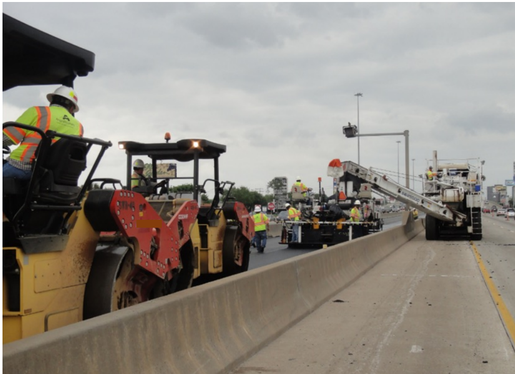
Figure 16. IH-69 overlay system construction. Source: Tom Scullion, TTI
