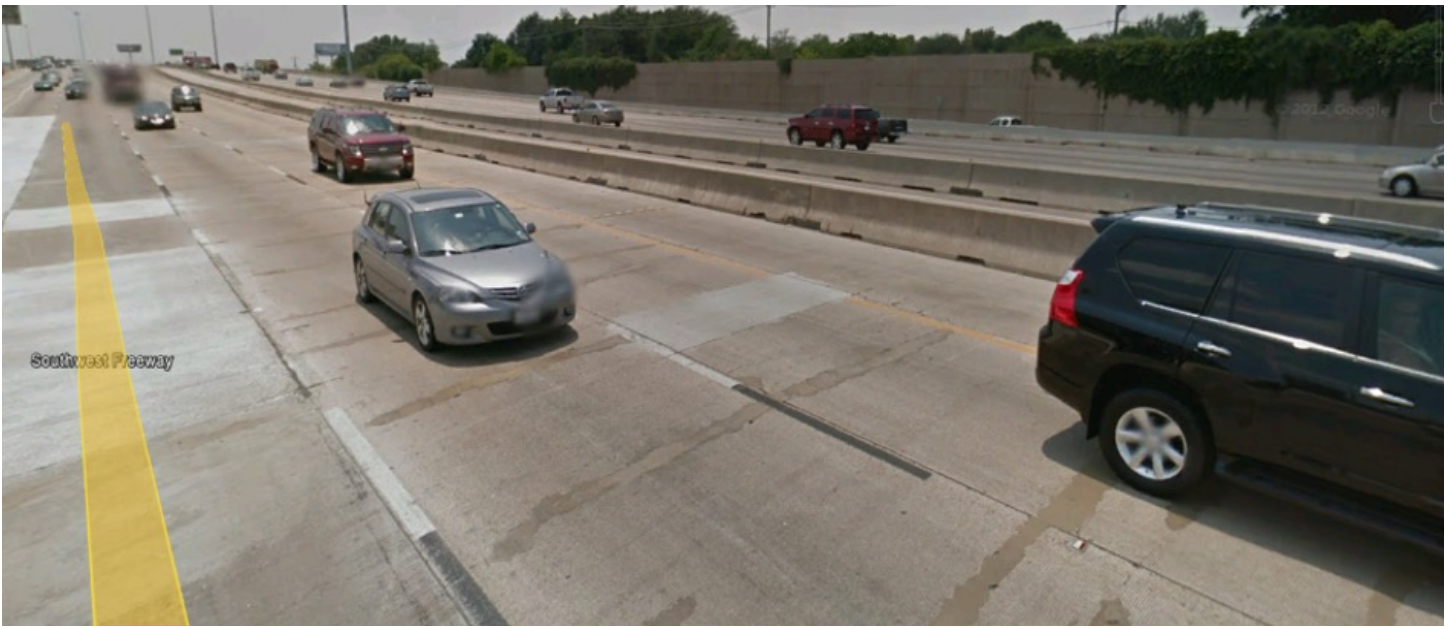
Figure 4. Existing surface repairs were made before rehabilitation. Source: Tom Scullion, TTI
