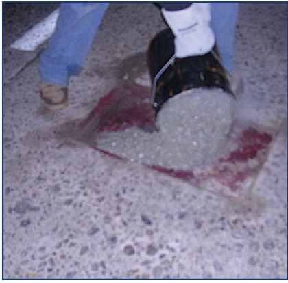
Figure 7. Spot repair. (Source: Blight 2021)
