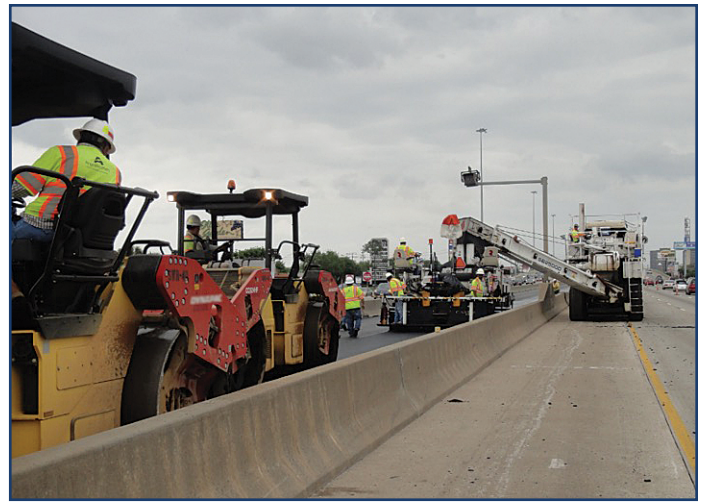
Figure 25. Use of MTV with tandem breakdown rollers. (Source: Tom Scullion, TTI)
