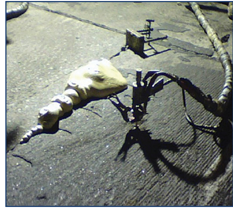
Figure 8. Slab stabilization using injection. (Source: Blight 2021)
