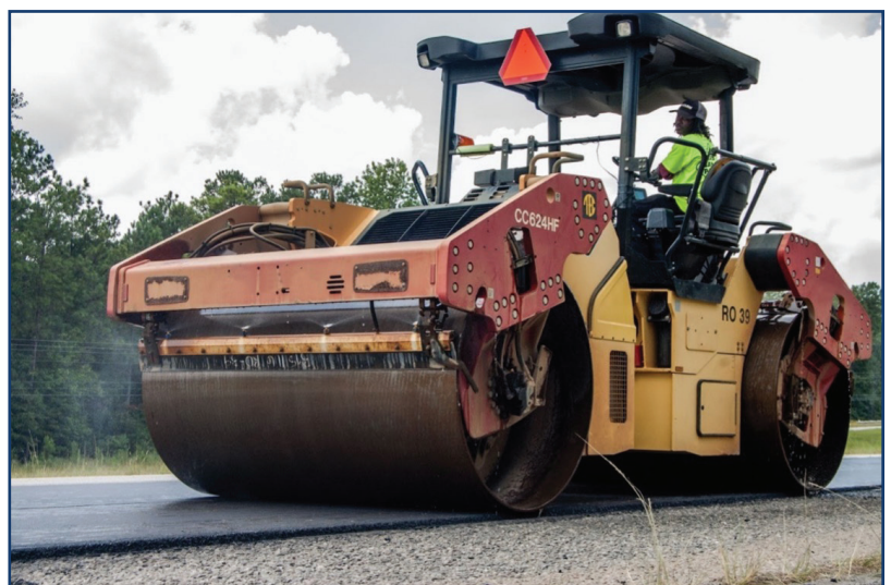
Figure 17. HPTO compaction. (Source: NCAT)
