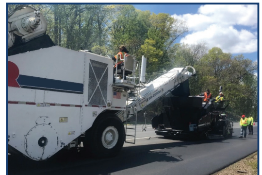
Figure 15. Use of MTV and spray-paver with a hopper insert. (Source: NJDOT)
