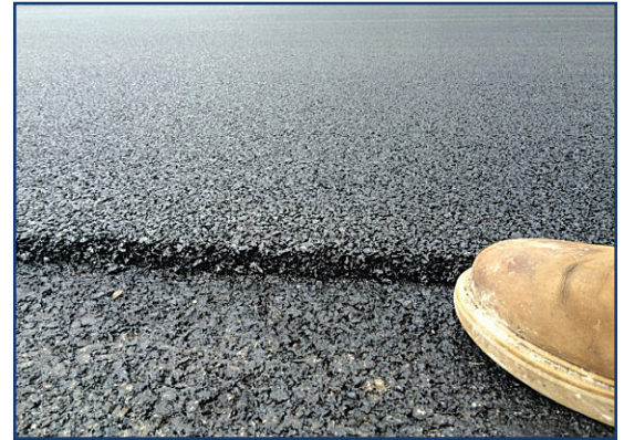
Figure 1. Finished HPTO surface. (Source: NCAT)
