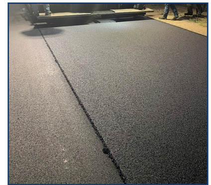
Figure 3. Freshly placed, uncompacted HPTO. (Source: NJDOT)
