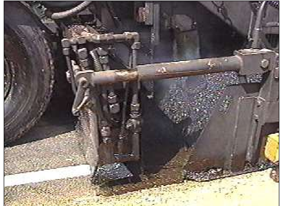
Spray Paver – Emulsion and HMA in one pass
