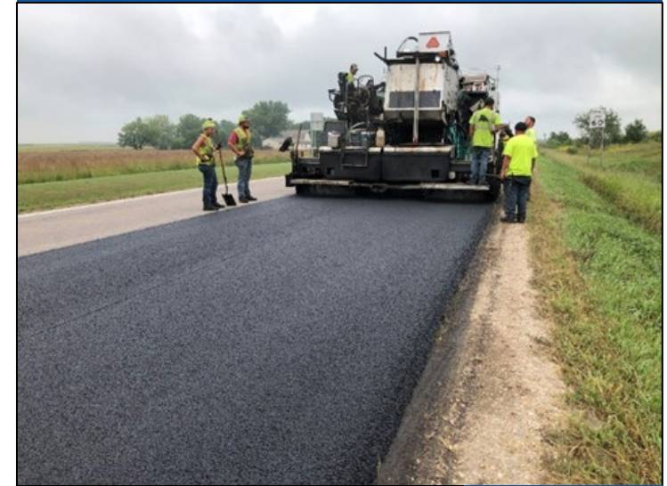
Newly Paved Ultra-Thin Bonded Wearing Coarse (UTBWC) Section
