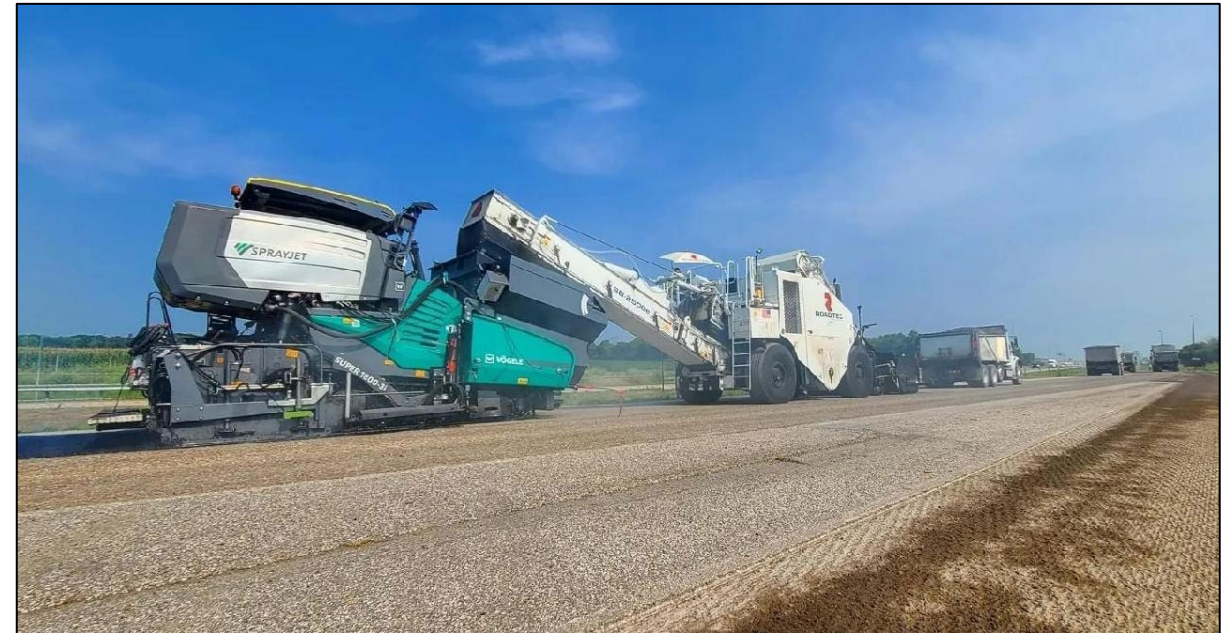
Material Transfer Vehicle (MTV) and Spray Paver
